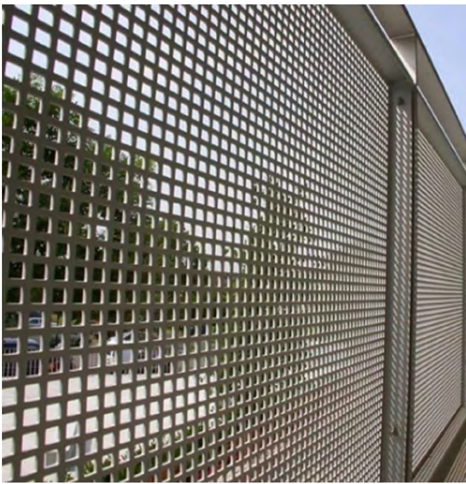
MECHANICAL SCREENING: PERFORATED METAL TO MATCH FASCIA
