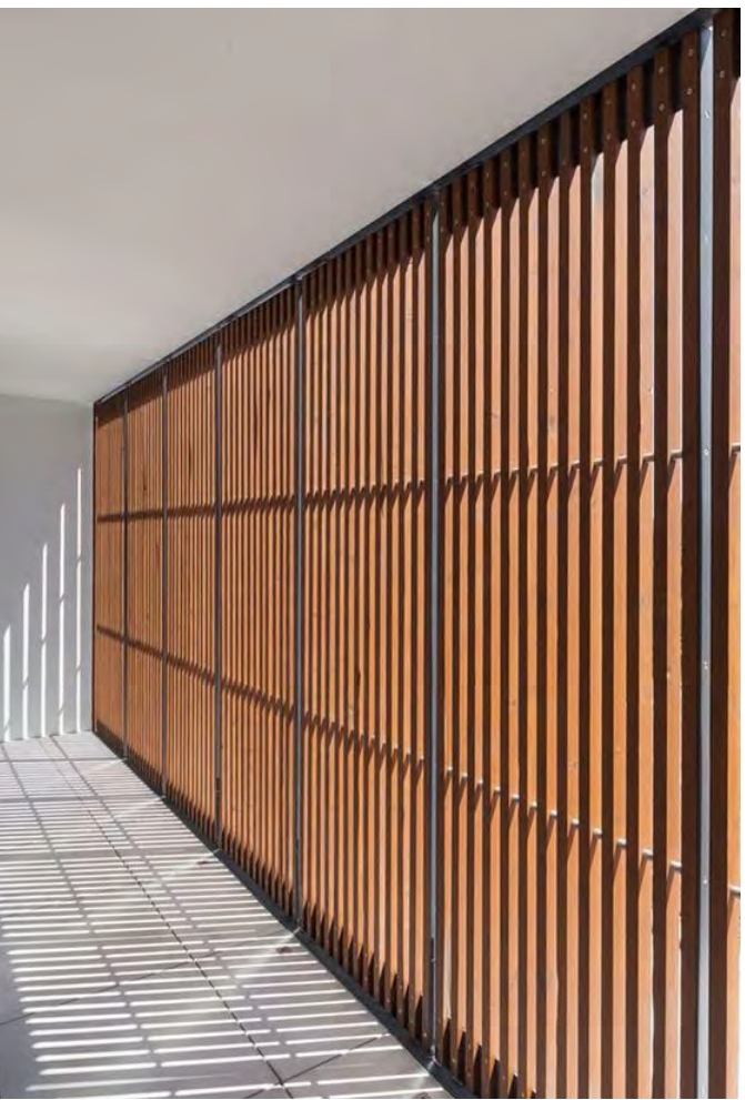
LOUVER SCREEN: THERMALLY MODIFIED WOOD
