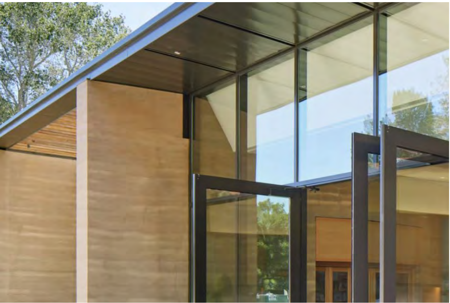
WINDOW/DOOR SYSTEM: THERMALLY BROKEN METAL/BLACK ANODIZED FINISH CLEAR GLASS: U-VALUE-.28 MIN./VLT-64% MIN.
