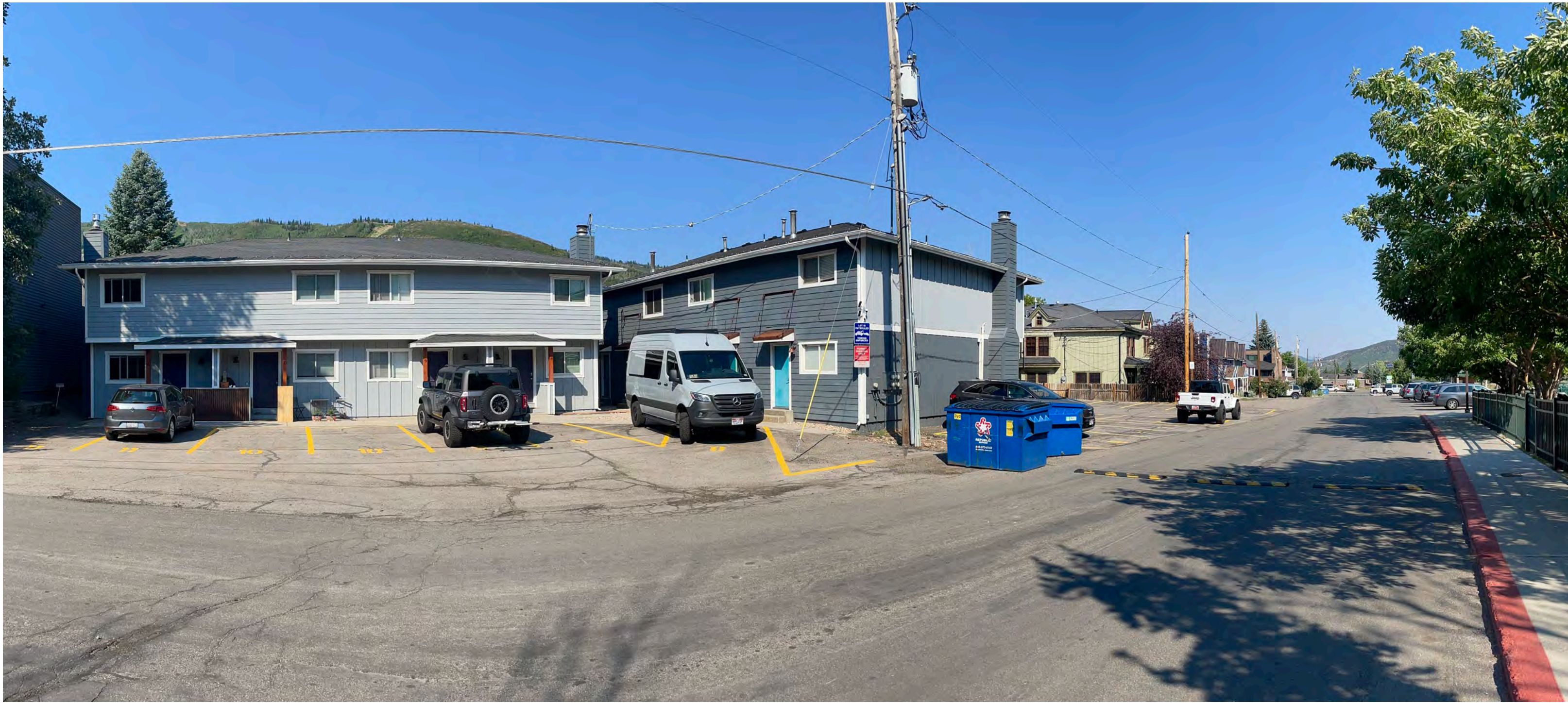
VIEW LOOKING NORTHWEST FROM SULLIVAN ROAD TOWARDS EXISTING CONDOMINIUMS
