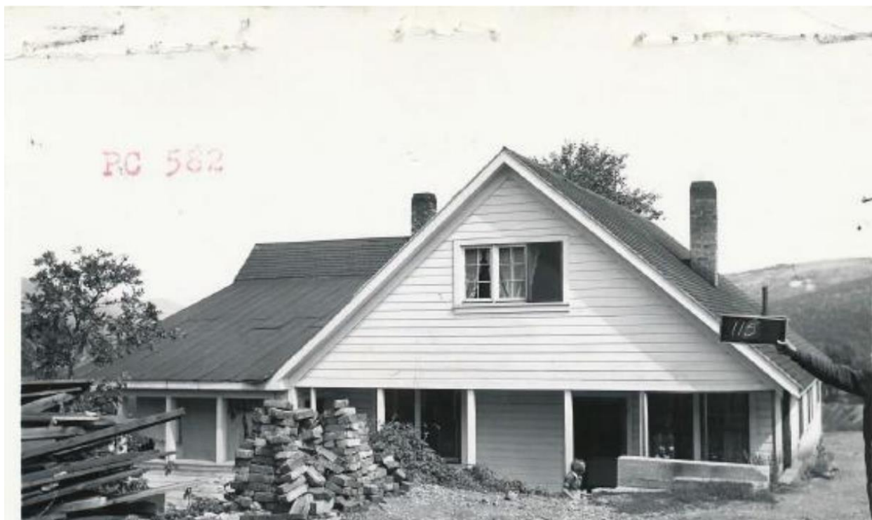
Figure 5: 1940s-era tax photo of 218 Sandridge Road, taken from the Historic Site Form.
