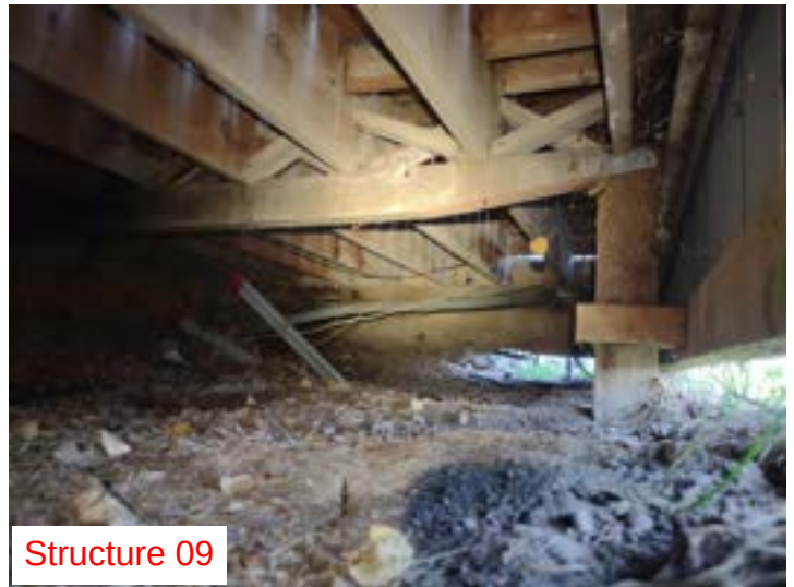
Wood joist structure of front porch.
