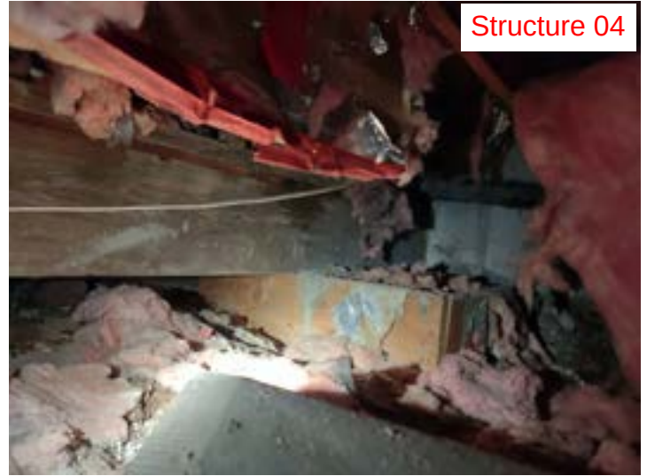
Floor joist sitting on CMU block and concrete spot footing at transition between historic and non-historic portion of house.
