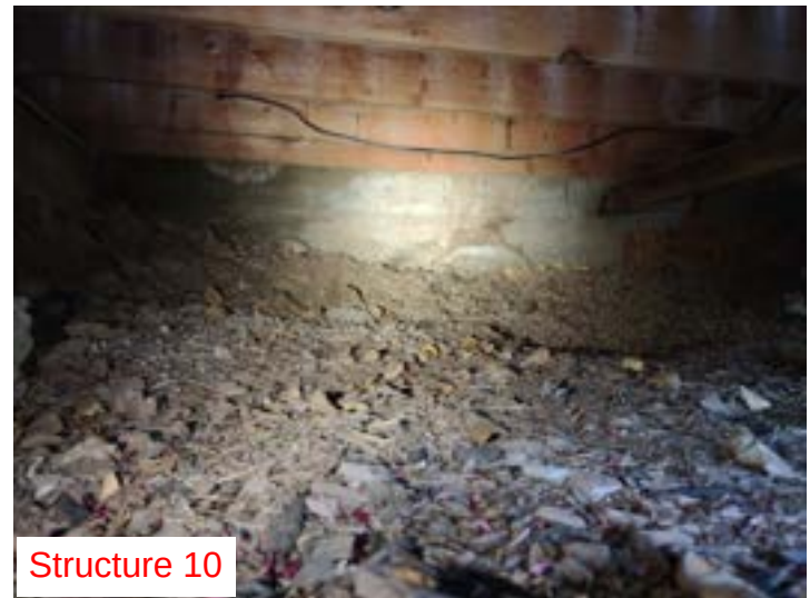
Wood joist structure of front porch, and area of concrete foundation at Northwest corner of house.
