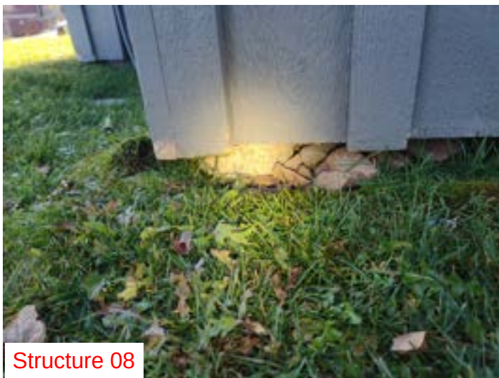
Concrete pier foundation on Northwest corner of front porch.
