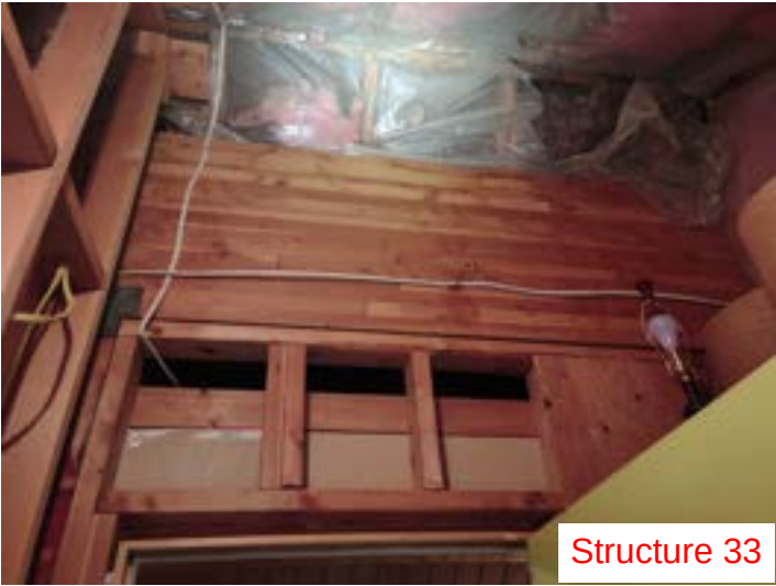
Vaulted roof framing Ridge beam for level 3 (1988 addition).
