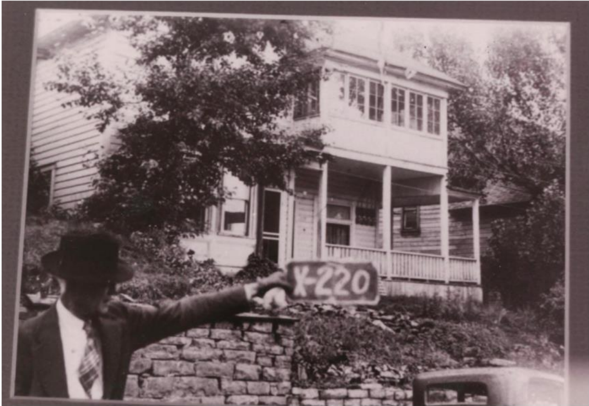
615 Woodside Avenue Tax Photo, circa 1941 showing the original sun room windows.
