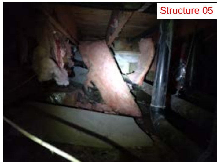
Floor joists tying into concrete foundation at non-historic back portion of house (1988 addition).
