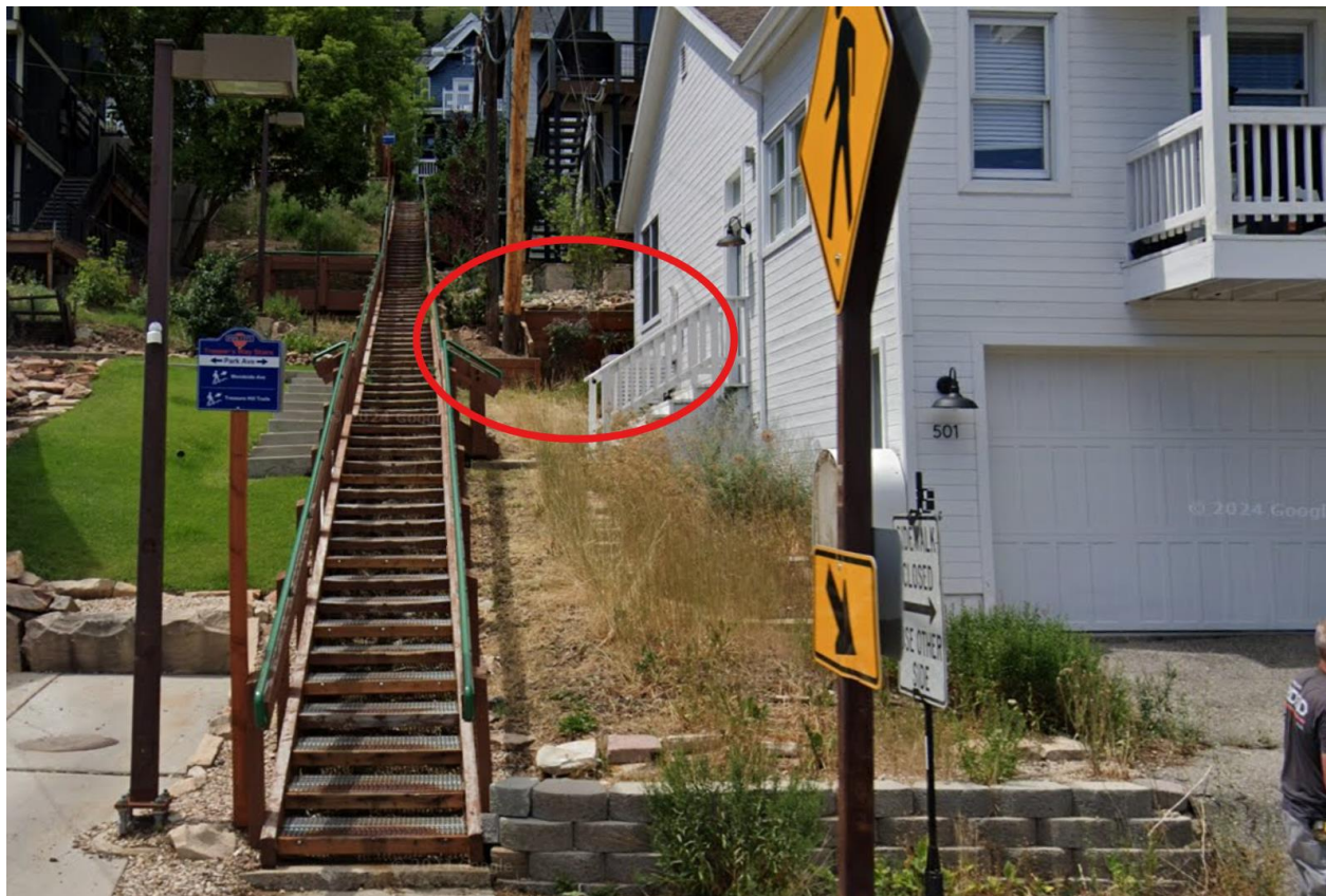
Figure 5: Google Maps photo showing visibility of the existing retaining wall at 501 Park Avenue from the Park Avenue Right-of-Way.
