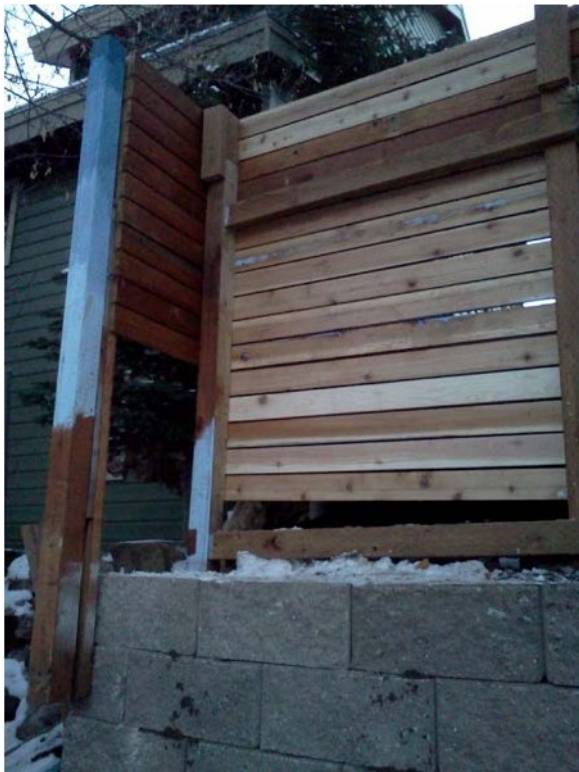
Poorly constructed fence, crooked. Ends still overhanging property line.
