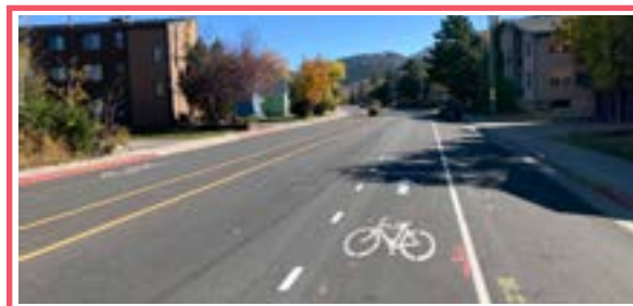
Park Ave Bike Lane & Shared Street | Deficient
