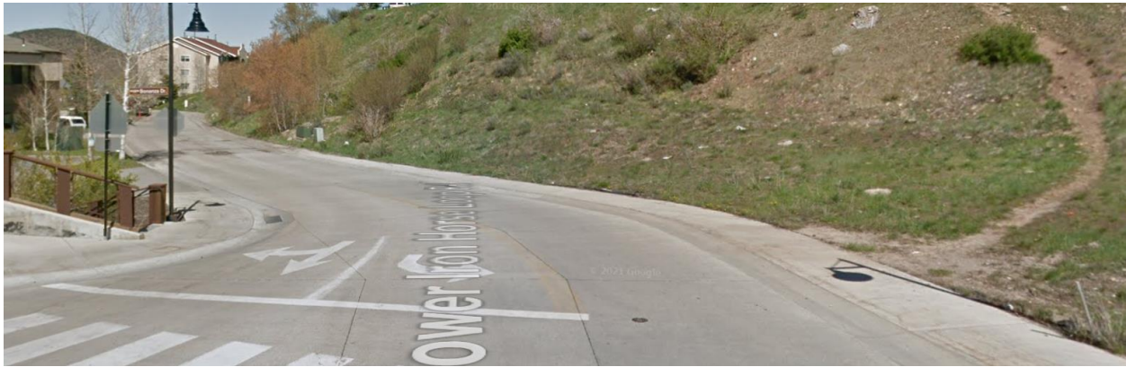
Parcel to the south of Lower Iron Horse Loop owned by Deer Valley that is a Steep Slope, possibly a Very Steep Slope. The Applicant proposes up to 20 Parking Spaces that require backing on to Lower Iron Horse Road and significant retaining walls.
