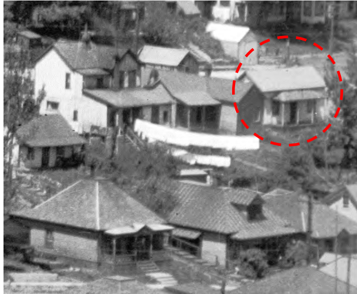
Figure 9: View of property at 424 Woodside in 1930, facing northwest. Note the retention of the simple hall-parlor form and addition of hip-roofed front porch, which was removed by 1941 according to the Sanborn Map. Photograph provided by Jonathan DeGray courtesy of Park City Historical Society and Museum.
