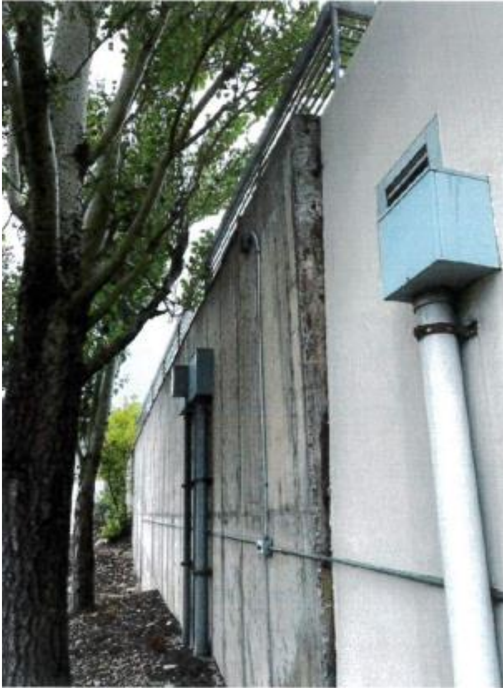
Figure 3: Image provided by Applicant showing the distance of the Retaining Wall southward from the City Hall foundation.
