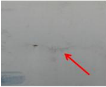
Figure 4: Fine crack
