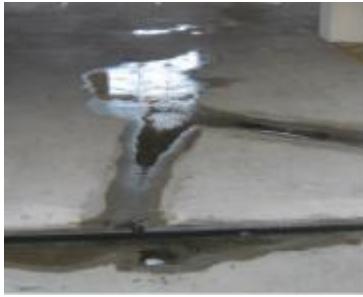
Figure 8: Ponding Water
