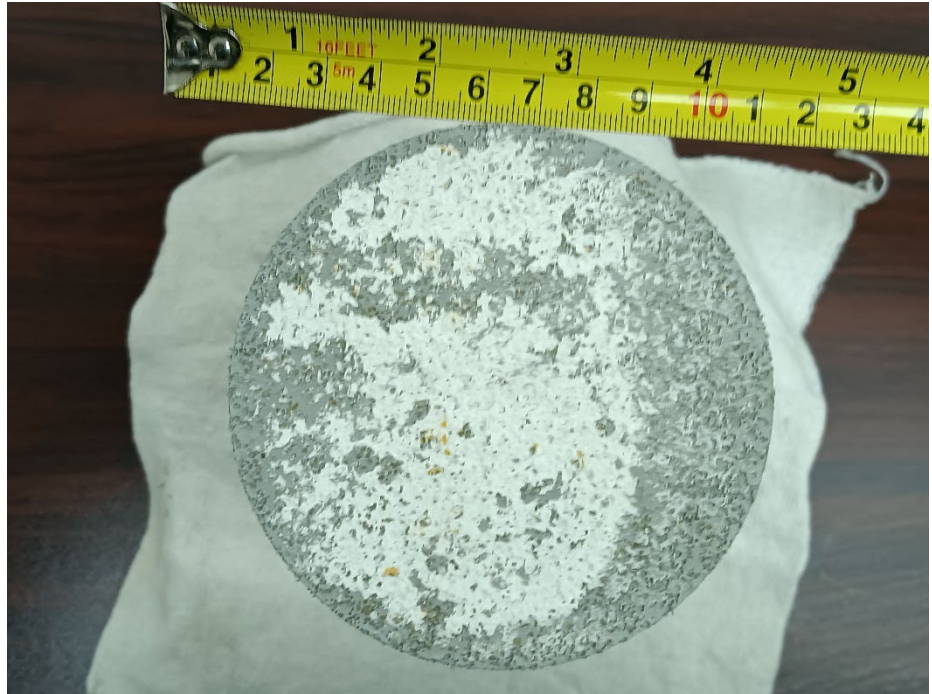
Photograph 3: Concrete core C-1 taken from the northwest corner of the upper deck of the parking structure.
