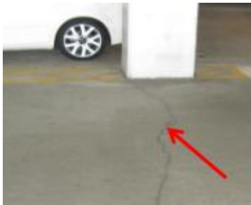
Figure 5: Medium Crack
