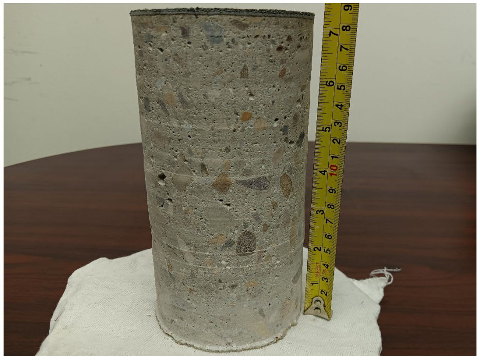
Photograph 12: Concrete core C-5 taken from the southwest portion of deck 3S in the parking structure.
