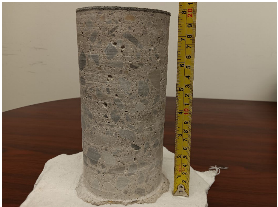
Photograph 4: Concrete Core C-1 taken from the northwest corner of the upper deck of the parking structure.
