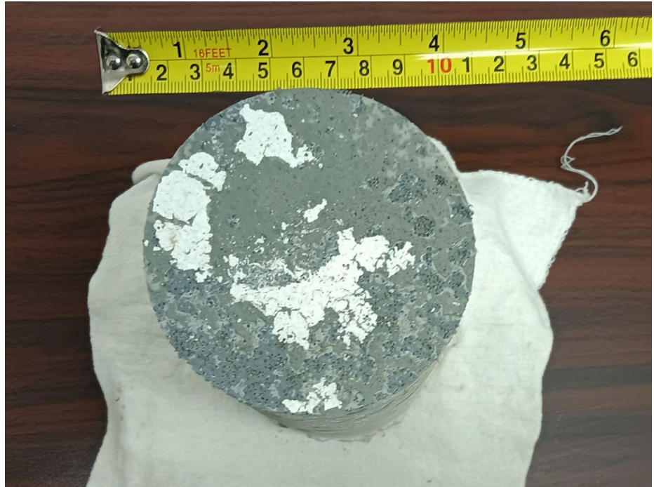
Photograph 5: Concrete core C-2 taken from the central portion of the upper deck of the parking structure.
