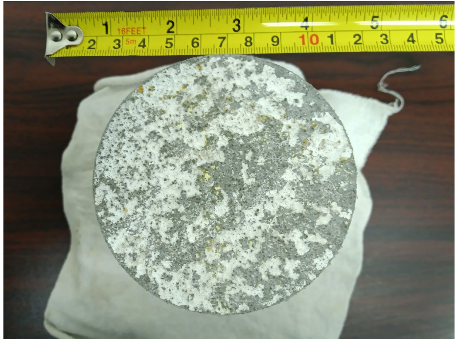
Photograph 9: Concrete core C-4 taken from the southwest portion of deck 3N in the parking structure.
