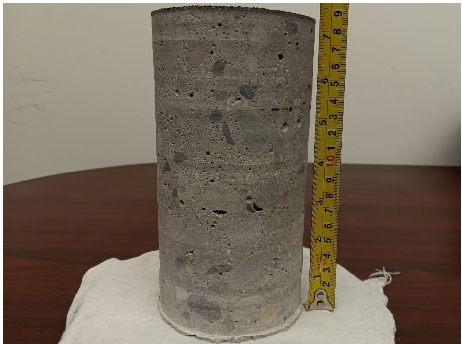
Photograph 16: Concrete core C-7 taken from the northwestern portion of deck 2S in the parking structure.
