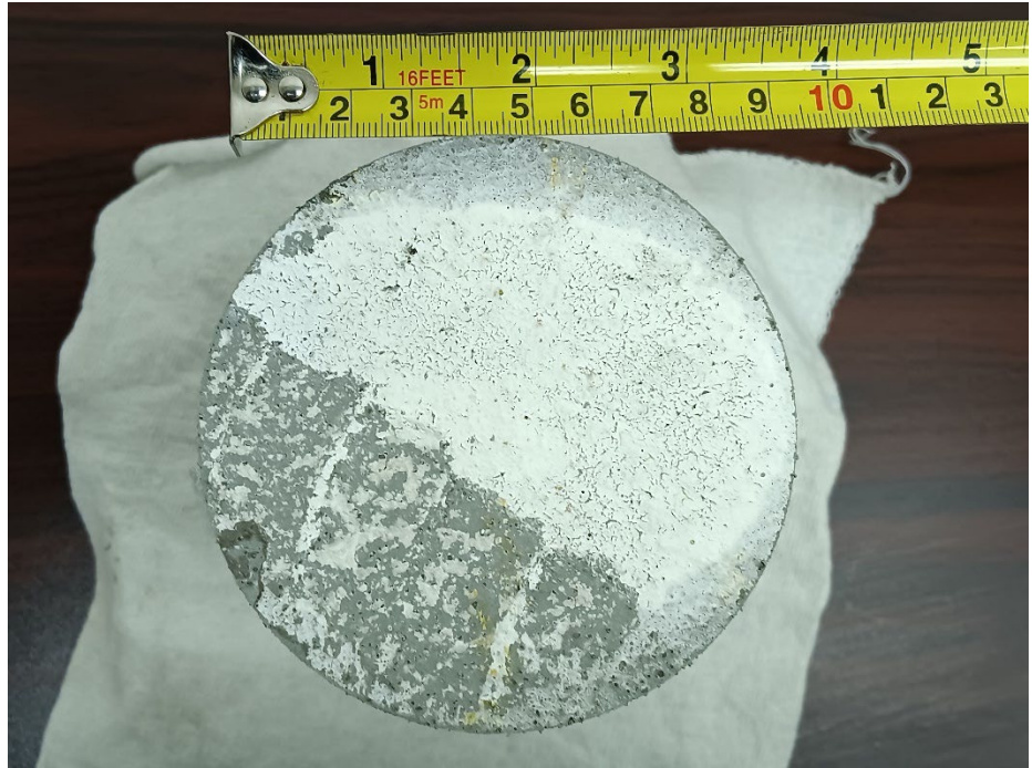
Photograph 17: Concrete core C-8 taken from the southeast portion of deck 2S in the parking structure.
