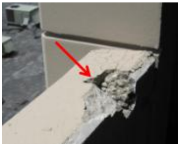
Figure 3: Concrete spall
