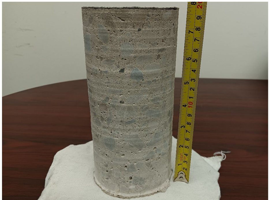
Photograph 10: Concrete core C-4 taken from the southwest portion of deck 3N in the parking structure.
