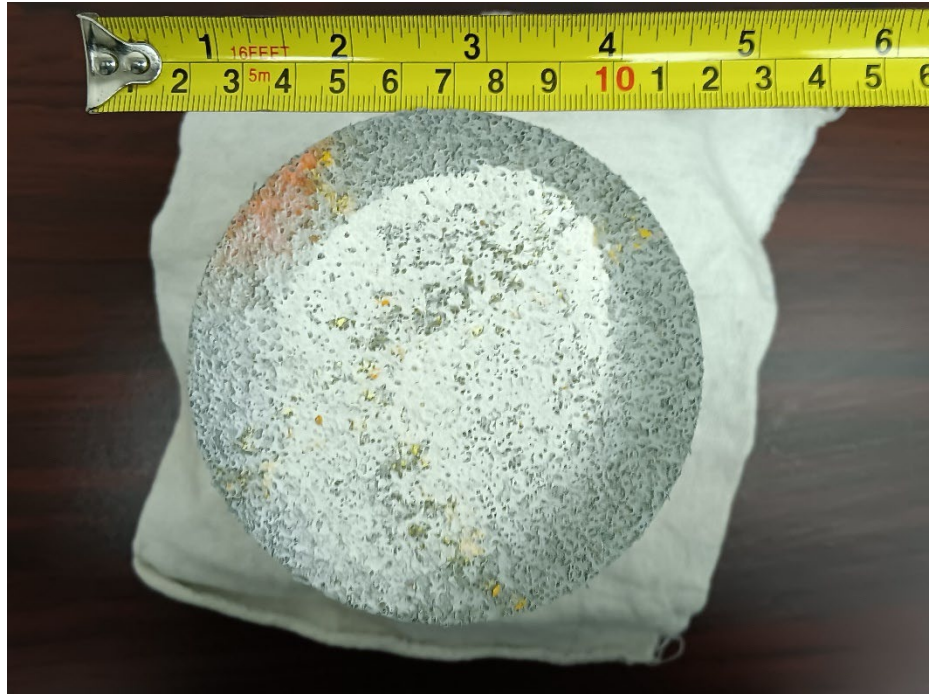
Photograph 7: Concrete core C-3 taken from the southwest corner of the upper deck of the parking structure.
