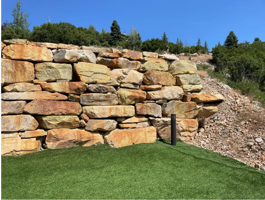
Figure 7: Retaining wall below the sports court and built within the Side Setback at 1115 Aerie Drive.
