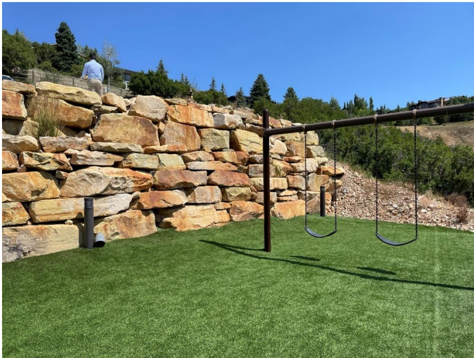
Figure 3: Retaining wall and astroturf playground area immediately south of the sports court and within the side Setback at 1115 Aerie Drive, pictured in July 2024.
