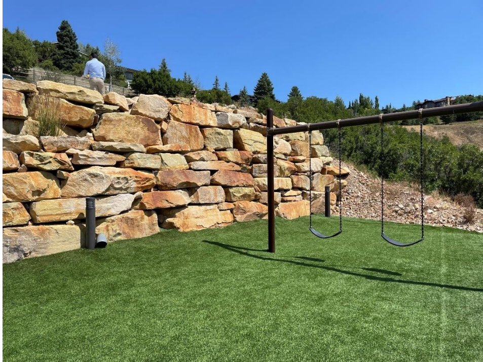
Figure 5: Retaining wall below the sports court and within the Side Setback at 1115 Aerie Drive.
