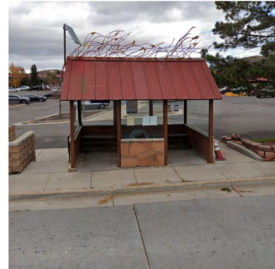
Existing Bus Stop, under Construction
