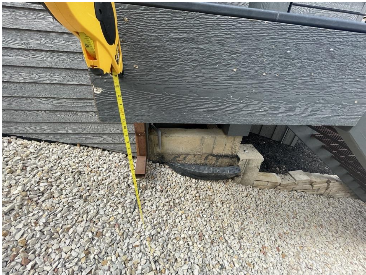
The Existing stairs, measured approximately 47" above Final Grade.
