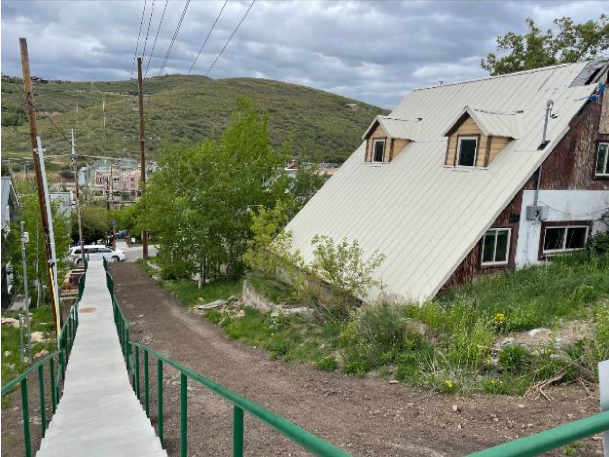
Figure 7: Public access stairs were constructed in the 9th Street right-of-way north of 844 Empire Avenue in 2024.
