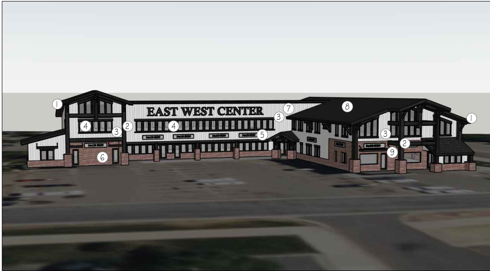
NORTH FRONT VIEW
