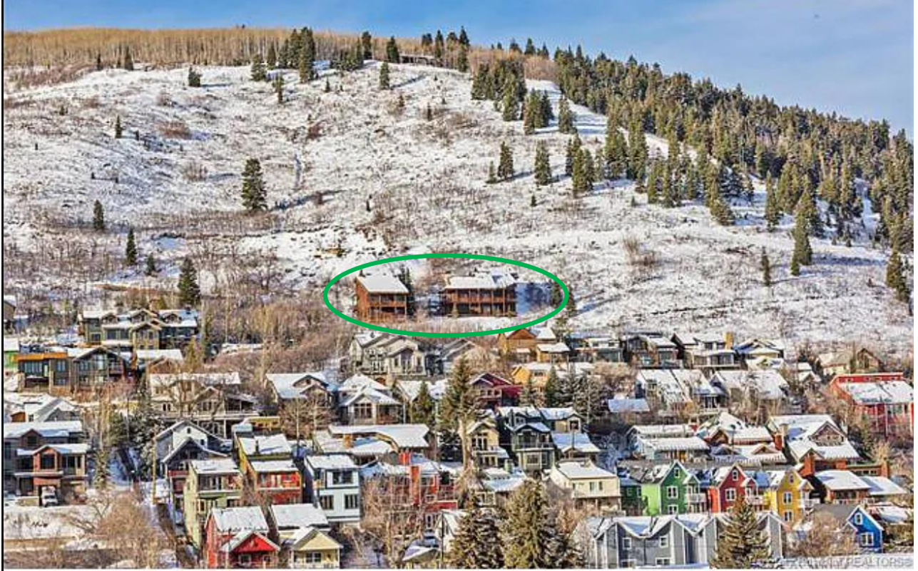
Figure 2: 220 King Road Single-Family Dwelling and Guest House, circled in green, recently demolished.
