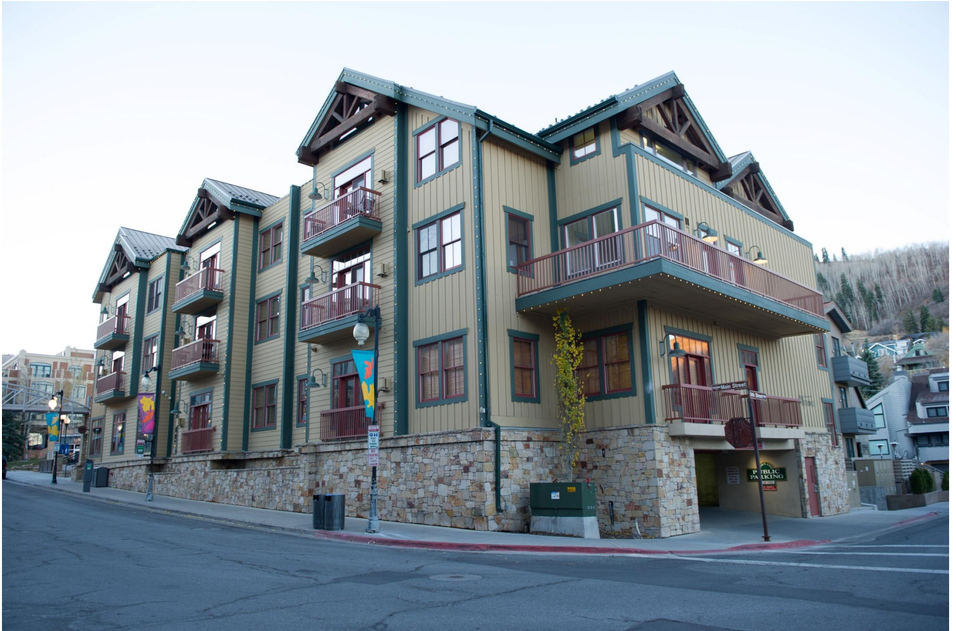
Lift Lodge At Town Lift - looking southerly
