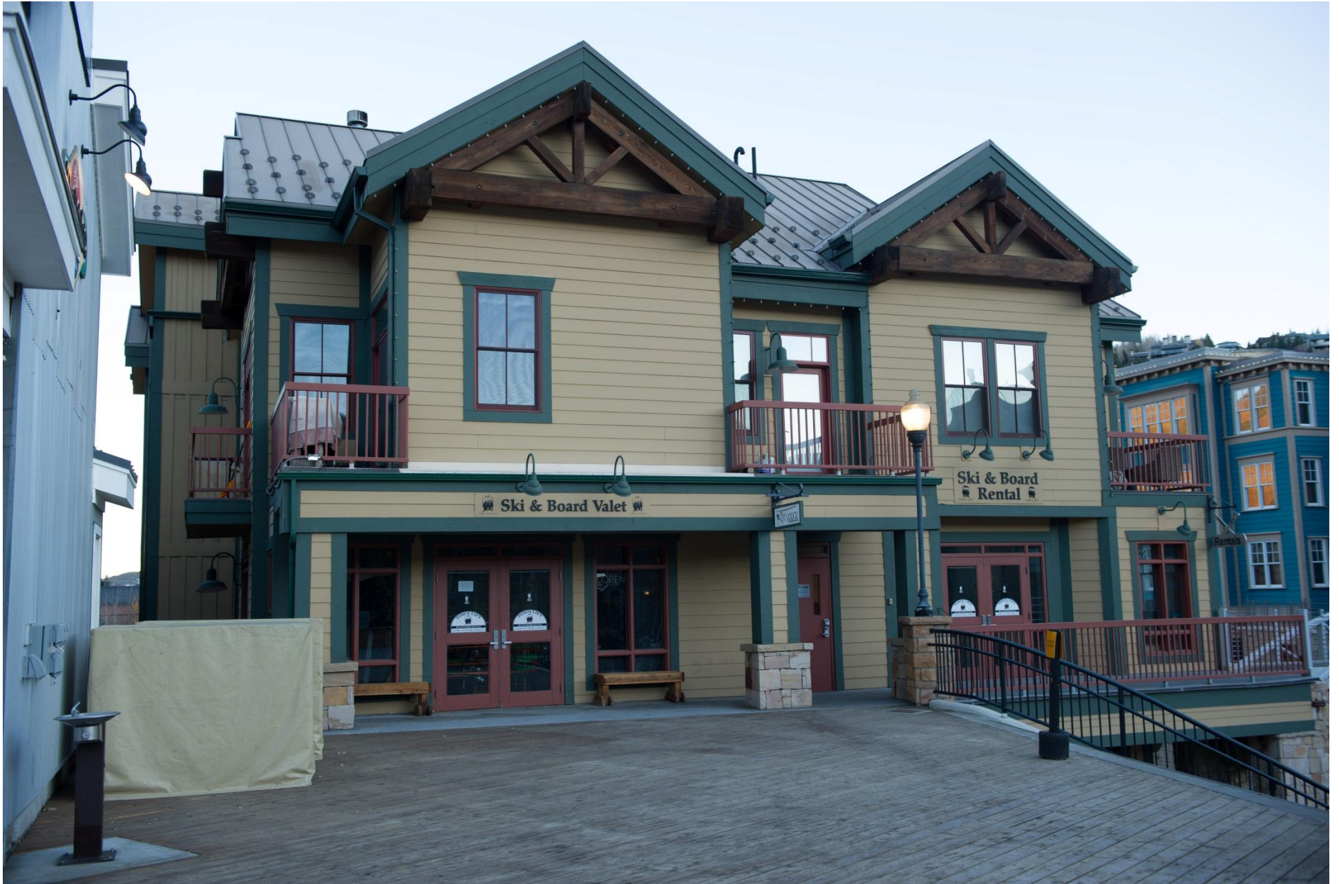
Lift Lodge At Town Lift - looking northerly
