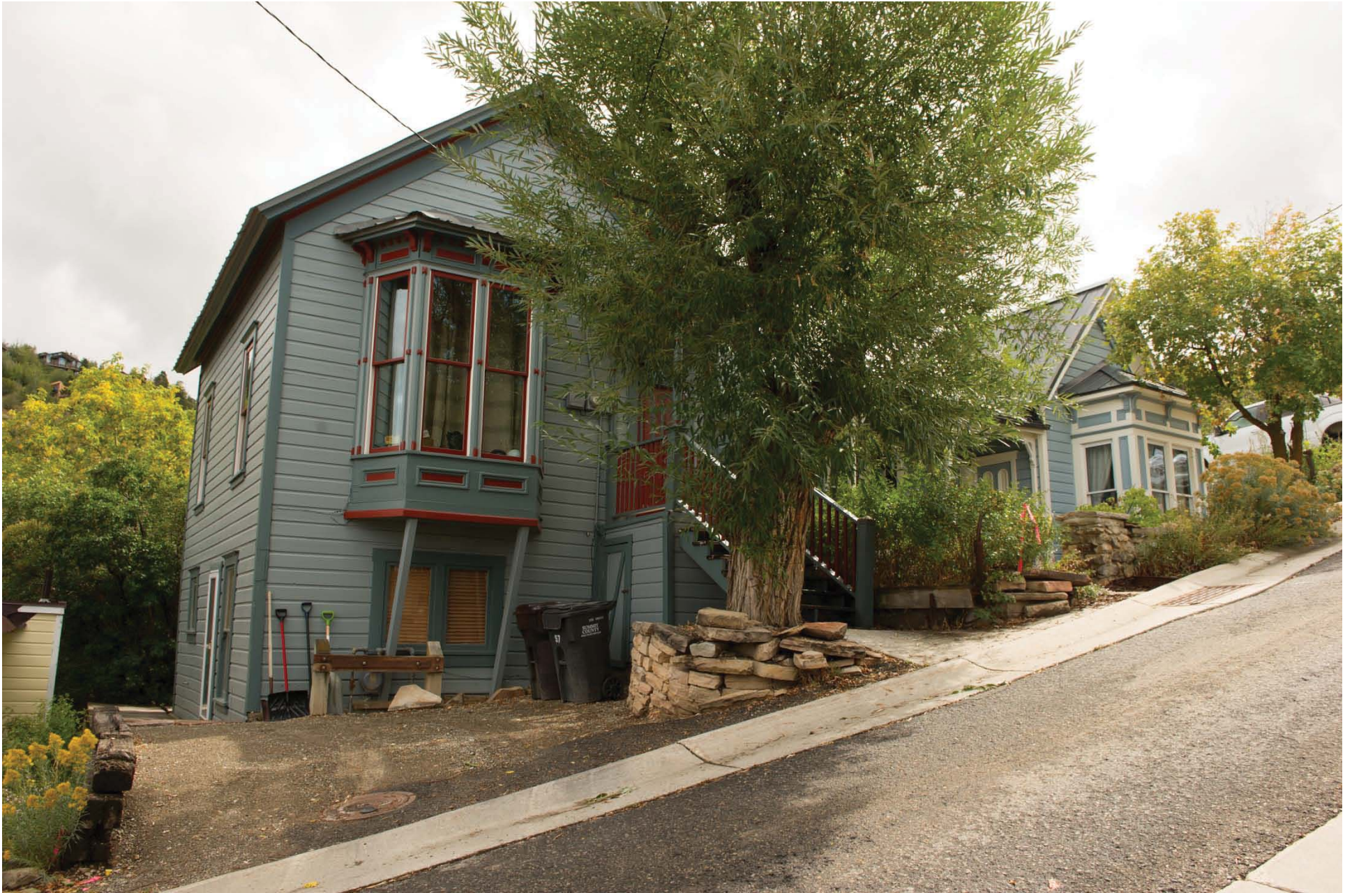
57 & 59 Prospect Street - looking easterly
