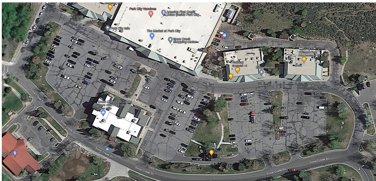
Figure 4: Existing Conditions Overview
