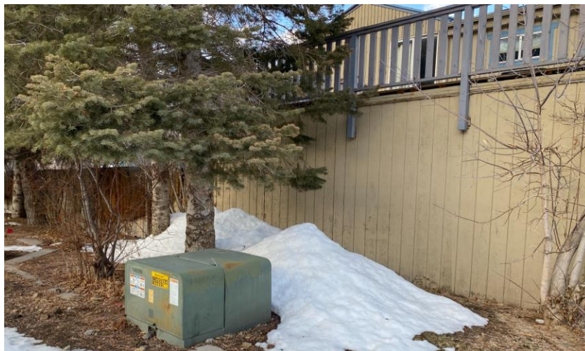
Image 1: On-site Photo of Rear Lot Line
