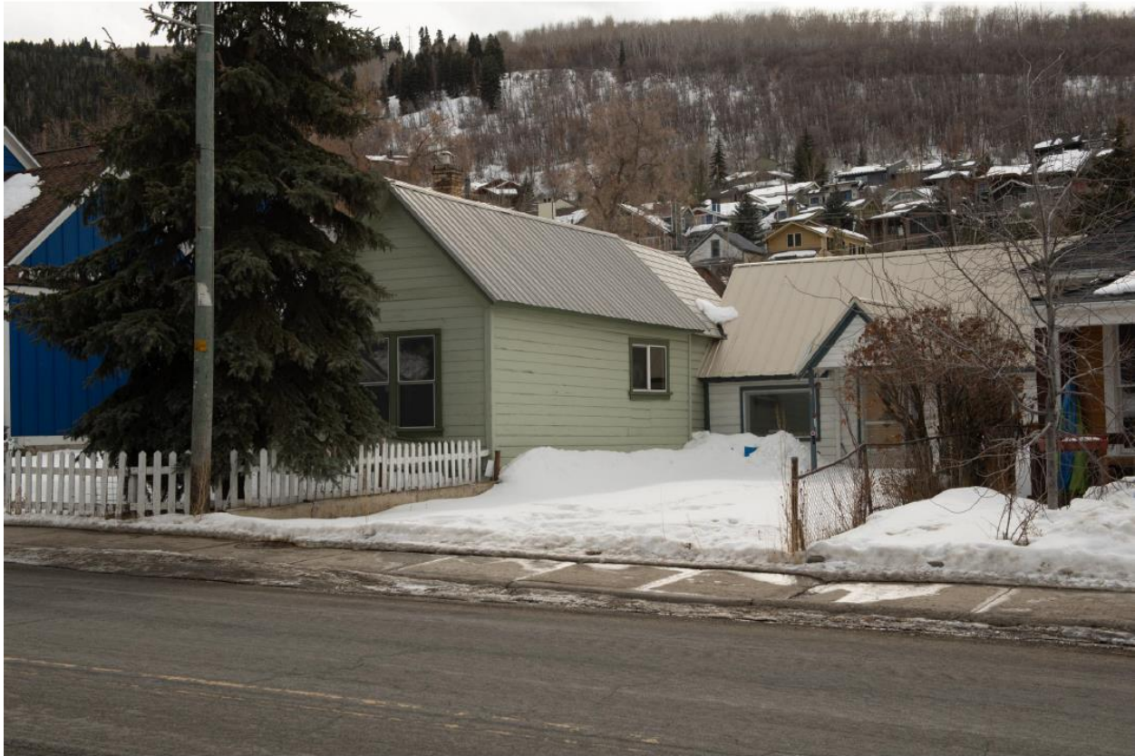
1125 (left) & 1129 (right) Park Avenue looking southerly
