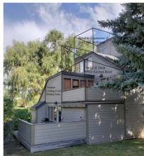
Decks Over Kitchen Area / Flat Roof Areas / Interior Vaulted Ceiling
