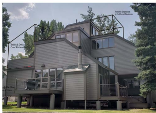
Tri-plex - Decks Over Kitchen Area / Flat Roof Area
