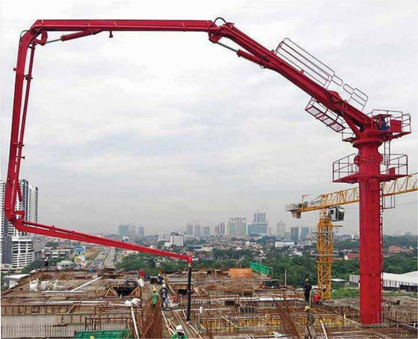
PLACING BOOM
