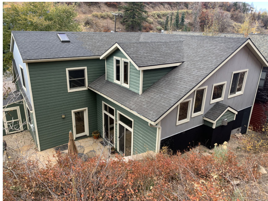
2. From SE Corner -showing existing wall & garage location
