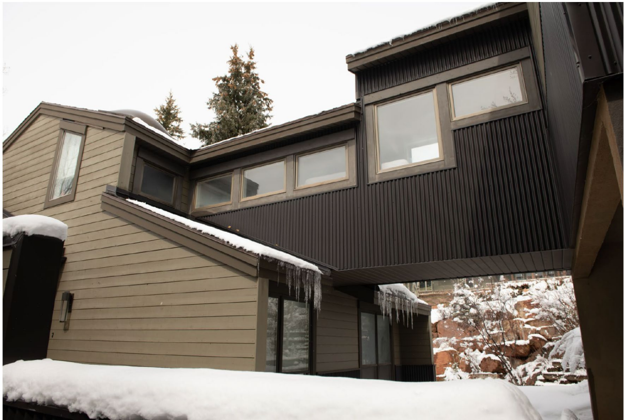
Figure 1 – 2587 Fairway Village Drive elevated walkway
