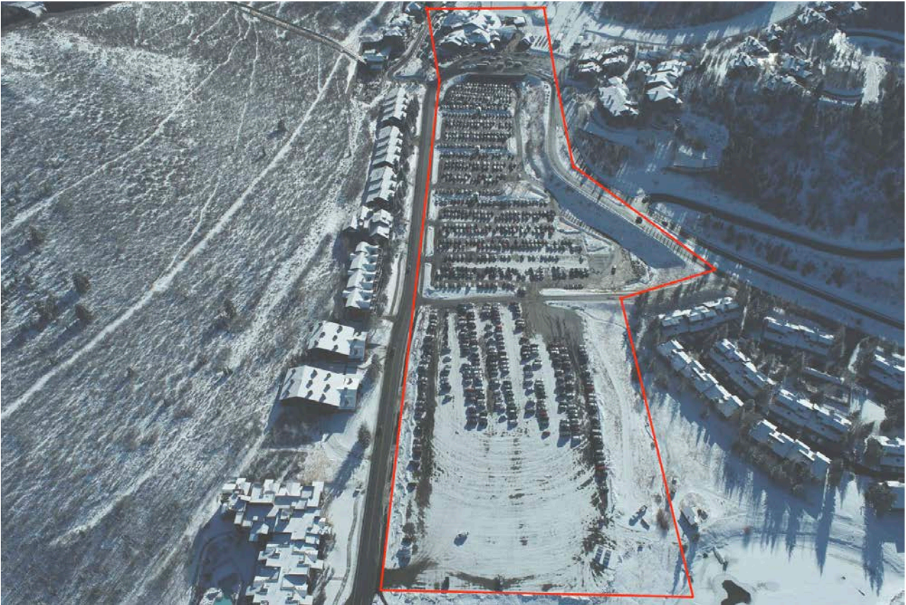
Existing Snow Park Village Development (outlined in red) looking south.
