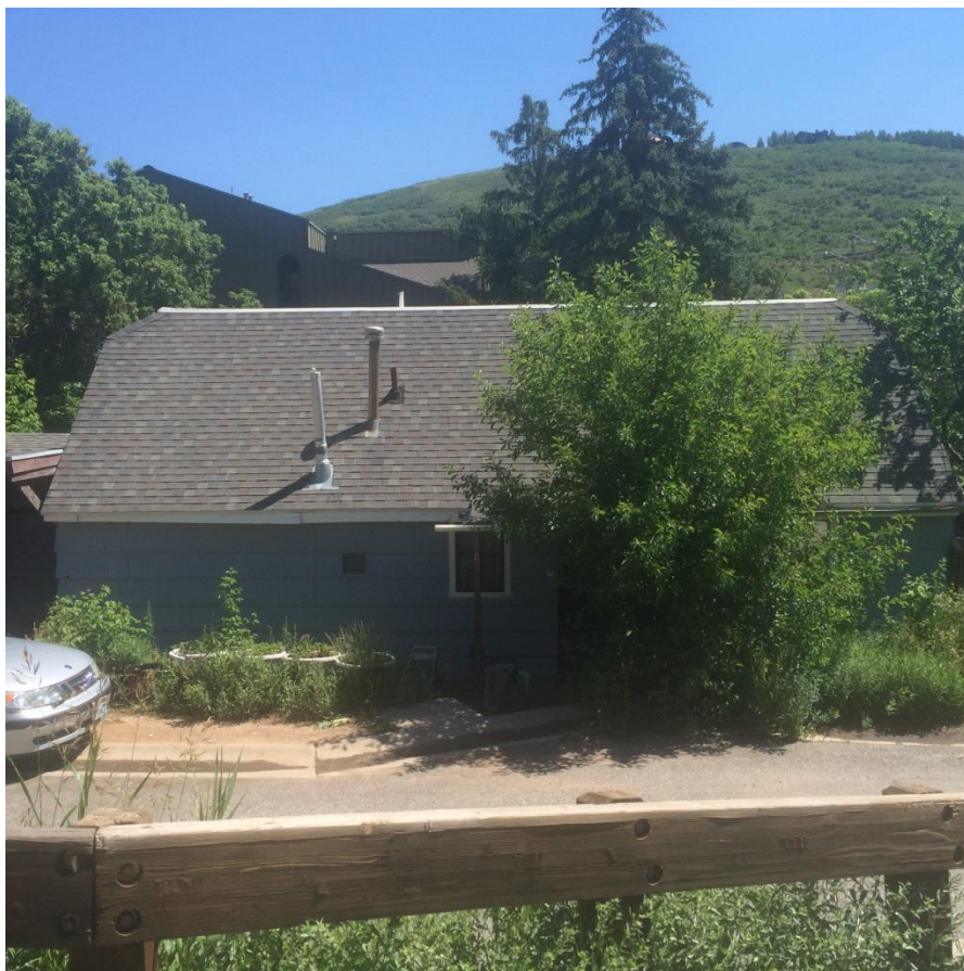
1302 Norfolk Avenue. West Elevation. June 2016.
