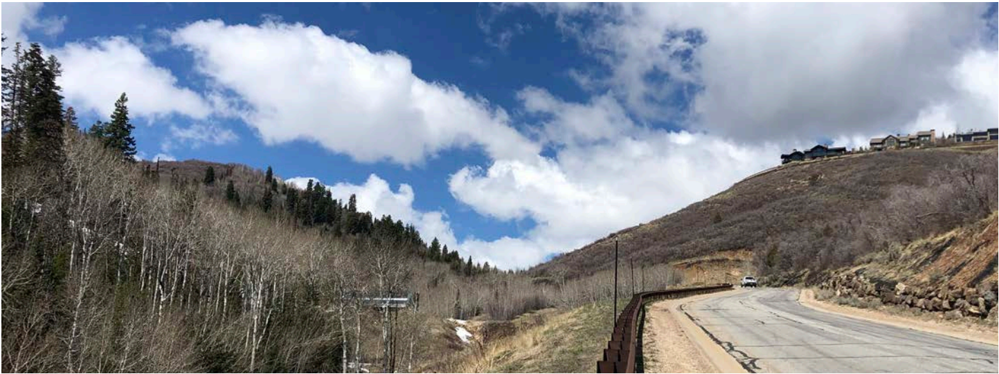
VIEW WEST UP DEER HOLLOW ROAD
