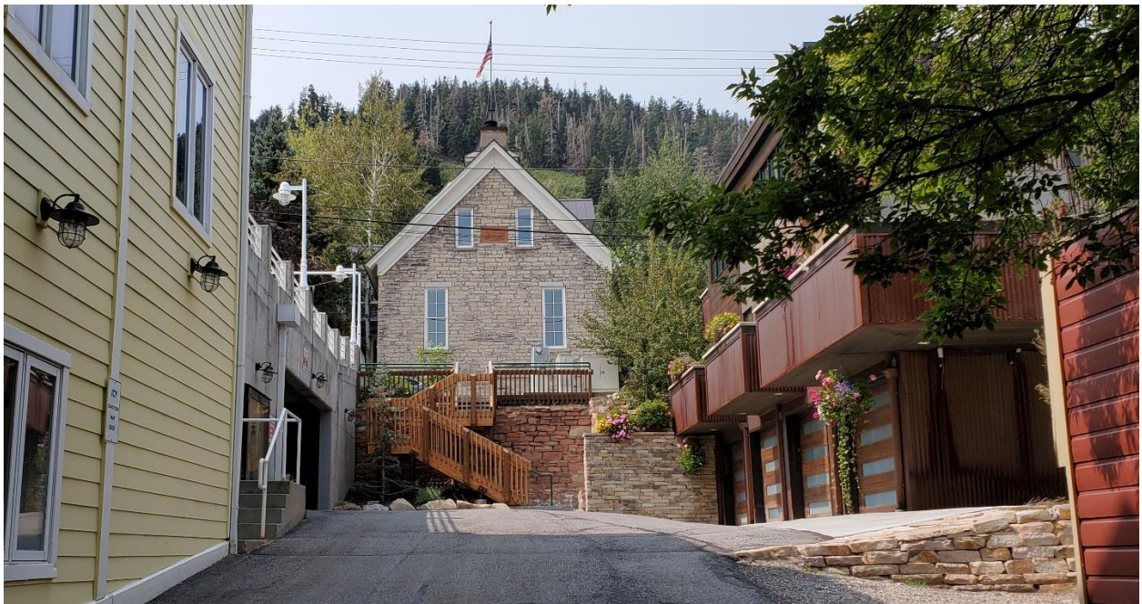
Figure 8. The Right-of-Way easement that provides access to the lower parking level
