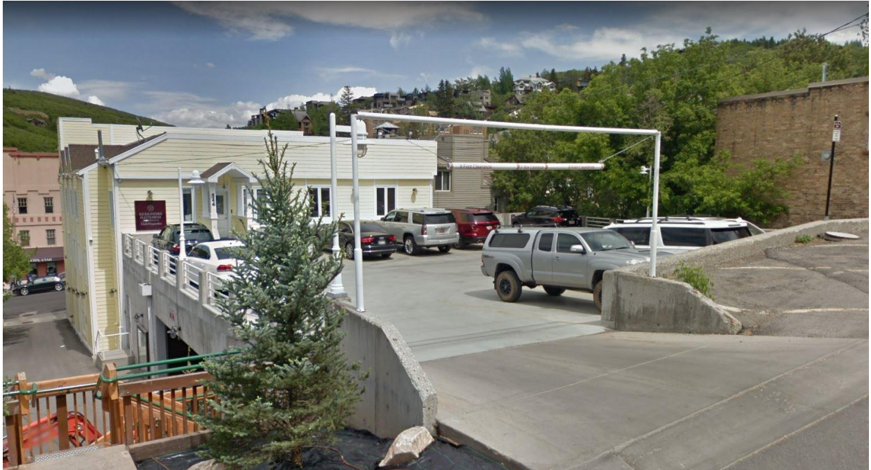
Figure 7. Upper level of the parking structure from Park Avenue
