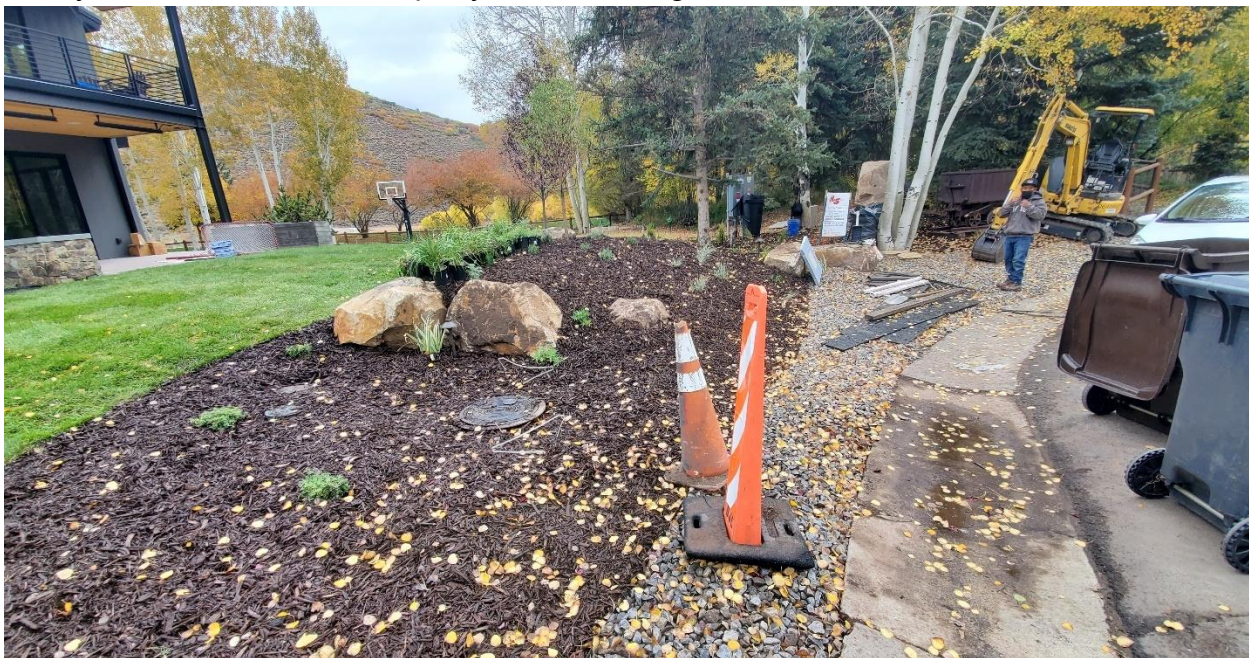
Figure 2: Looking east toward the Side Yard of the Property.
