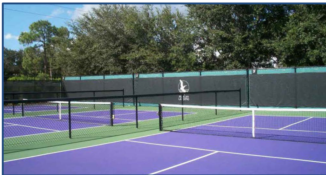
Figure 6. AcoustiFence Surrounding Pickleball Courts
