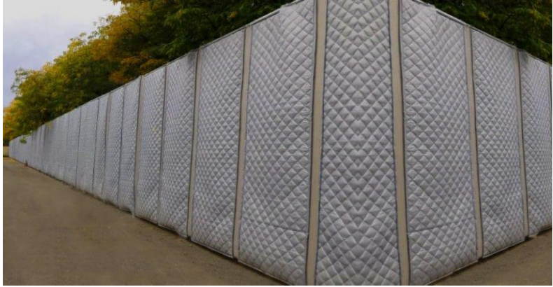
Figure 6. Illustration of pickleball courts with noise-mitigating fencing around the play area
