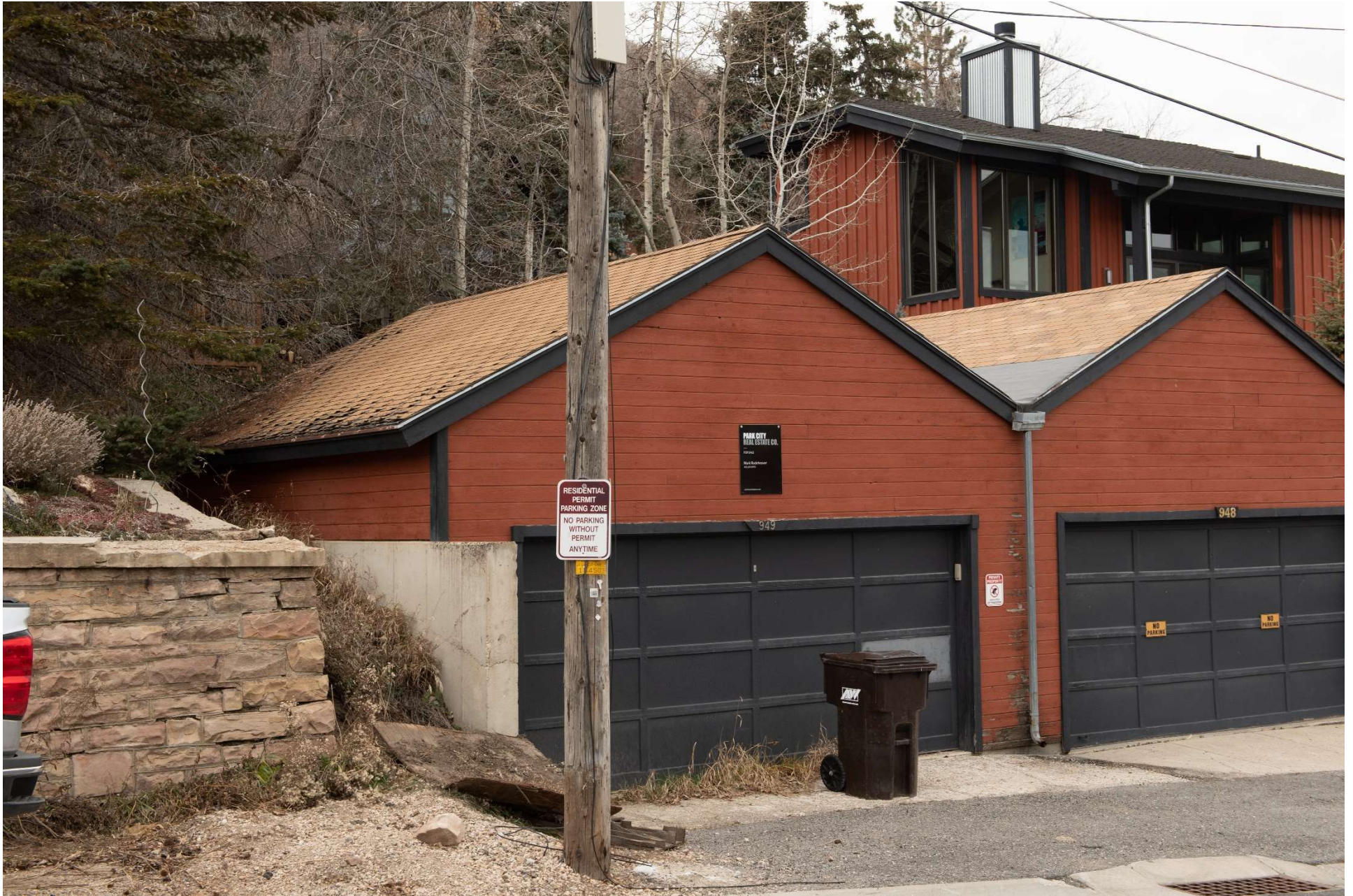
949 Empire Avenue - front - looking westerly
