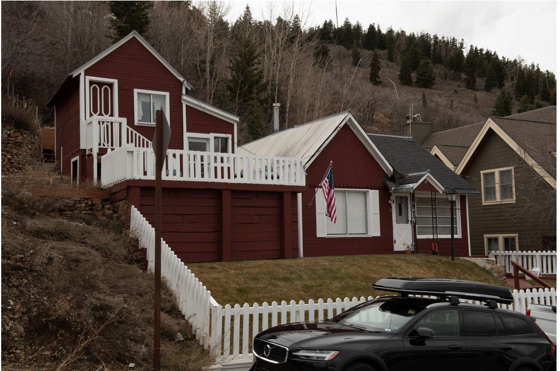
405 Woodside Avenue - front - looking west
