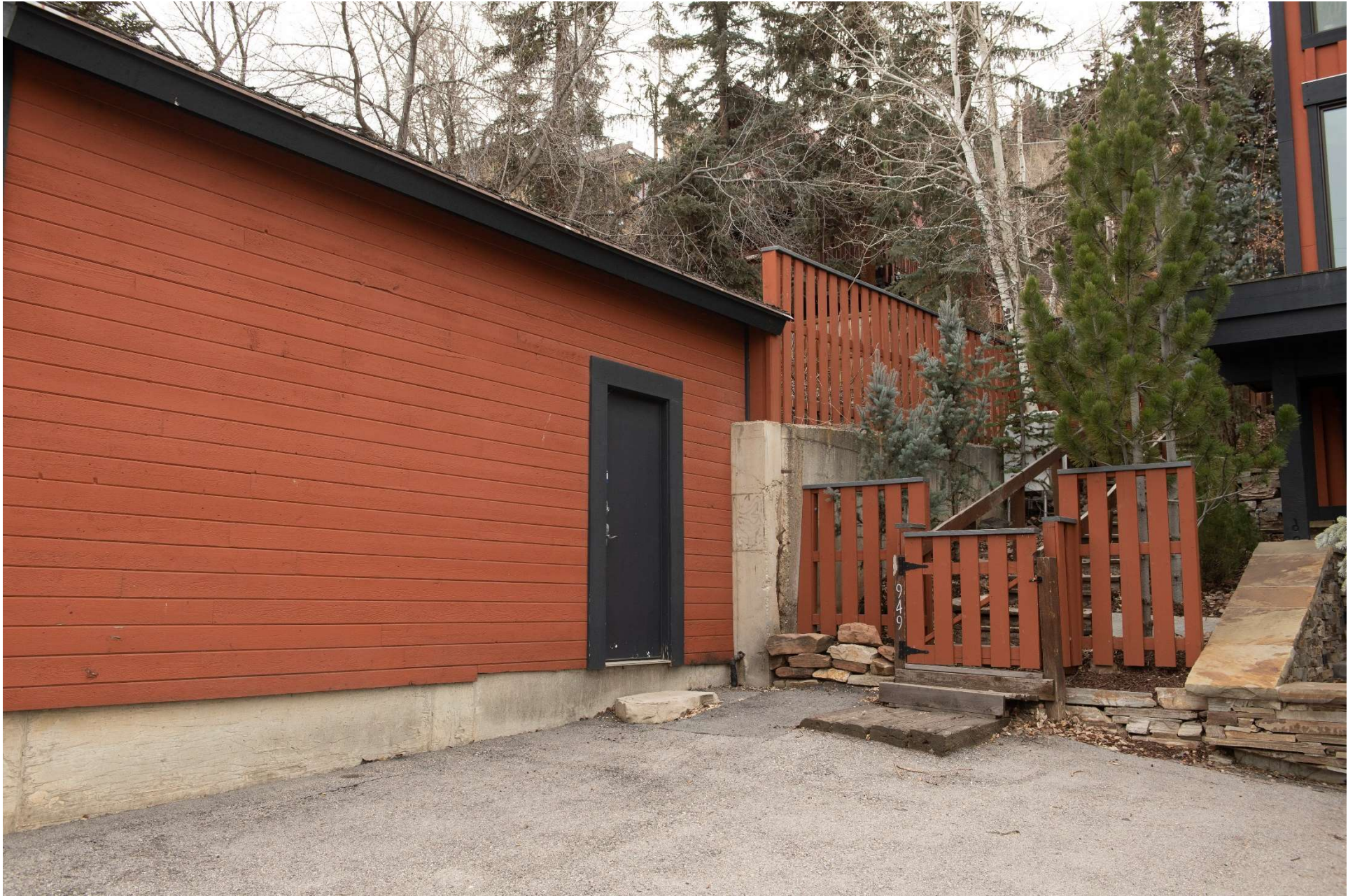
949 Empire Avenue - front - looking southwesterly
