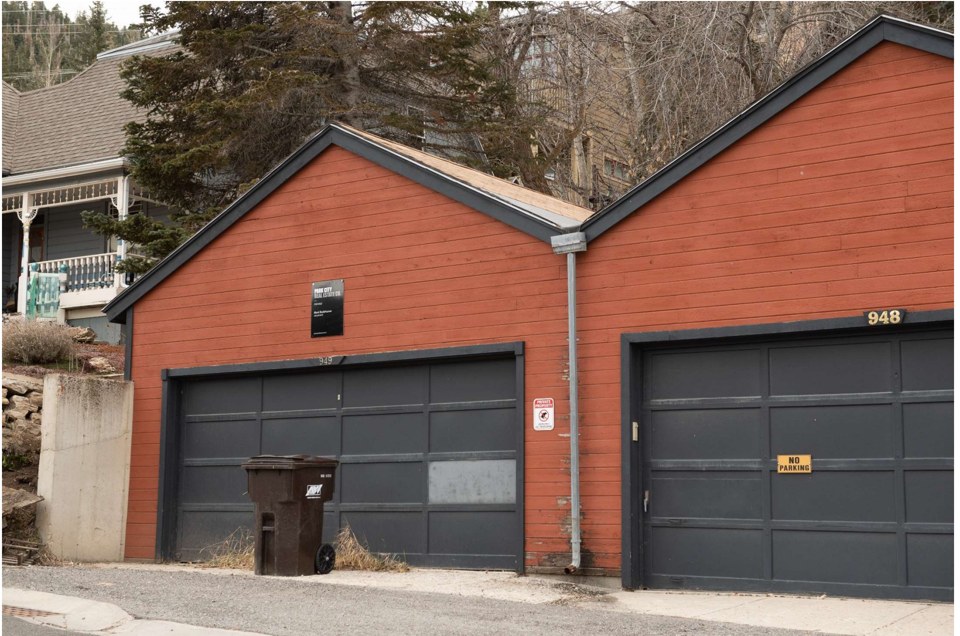
949 Empire Avenue - front - looking southwesterly
