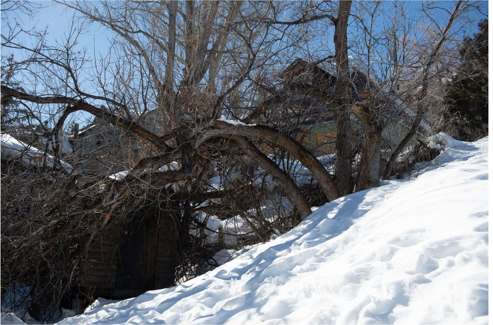
115 Sampson Ave - rear - looking southwesterly
