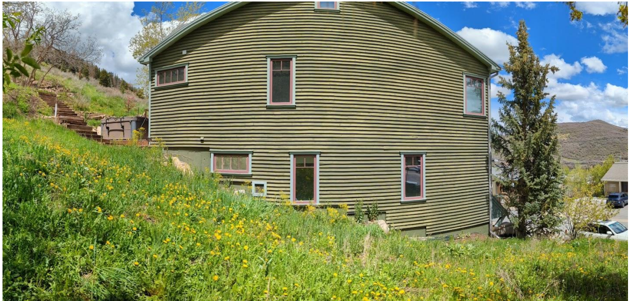
View from the South
