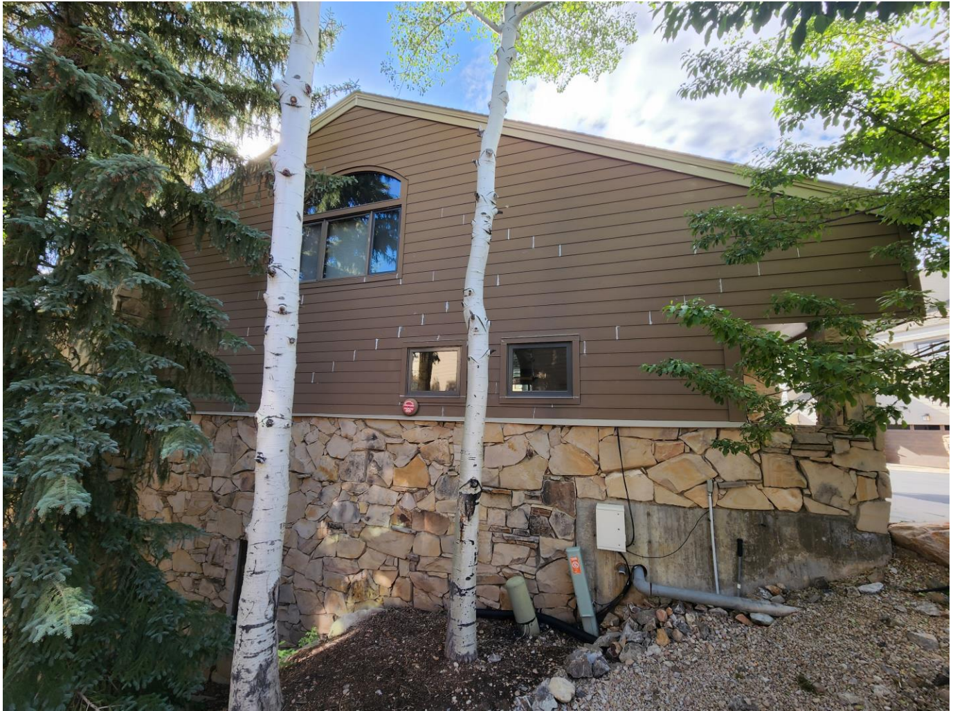
Unit 14F from the Southeast Corner of Unit 13F Looking Northeast
