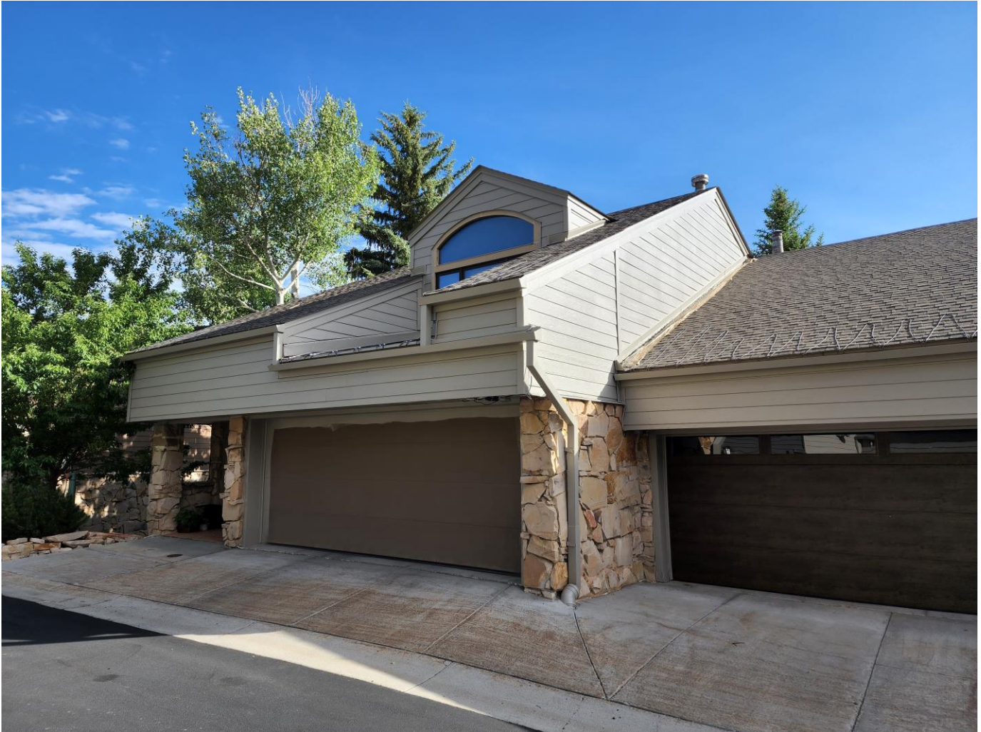
Unit 14F from Stonebridge Circle Looking Northwest
