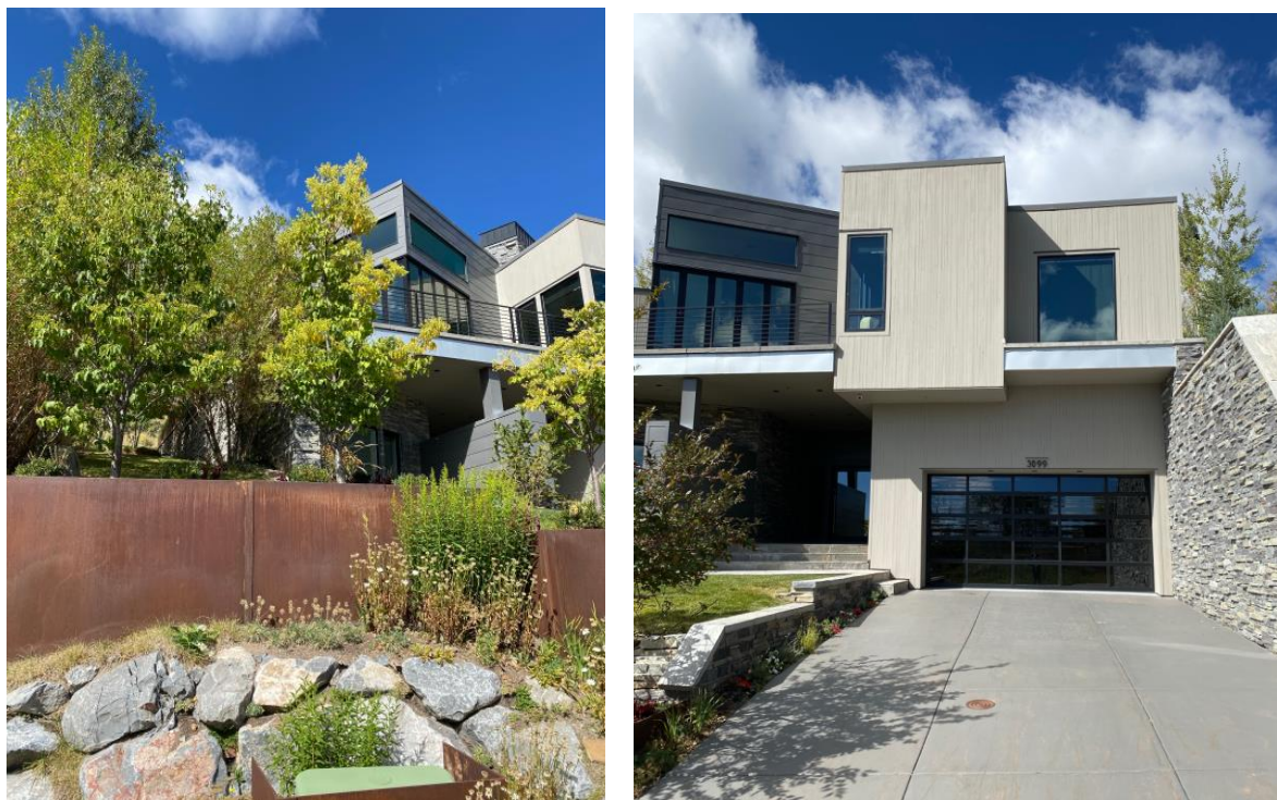
Figure 1: Front View of Applicant's Property
