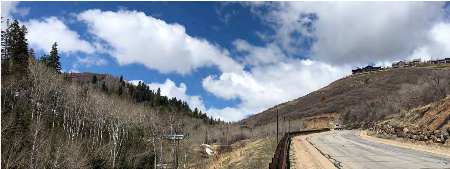
VIEW WEST UP DEER HOLLOW ROAD
