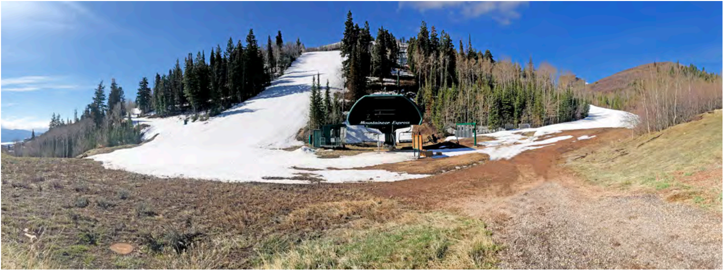
SITE VIEW LOOKING SOUTH TO MOUNTAINEER EXPRESS LIFT
