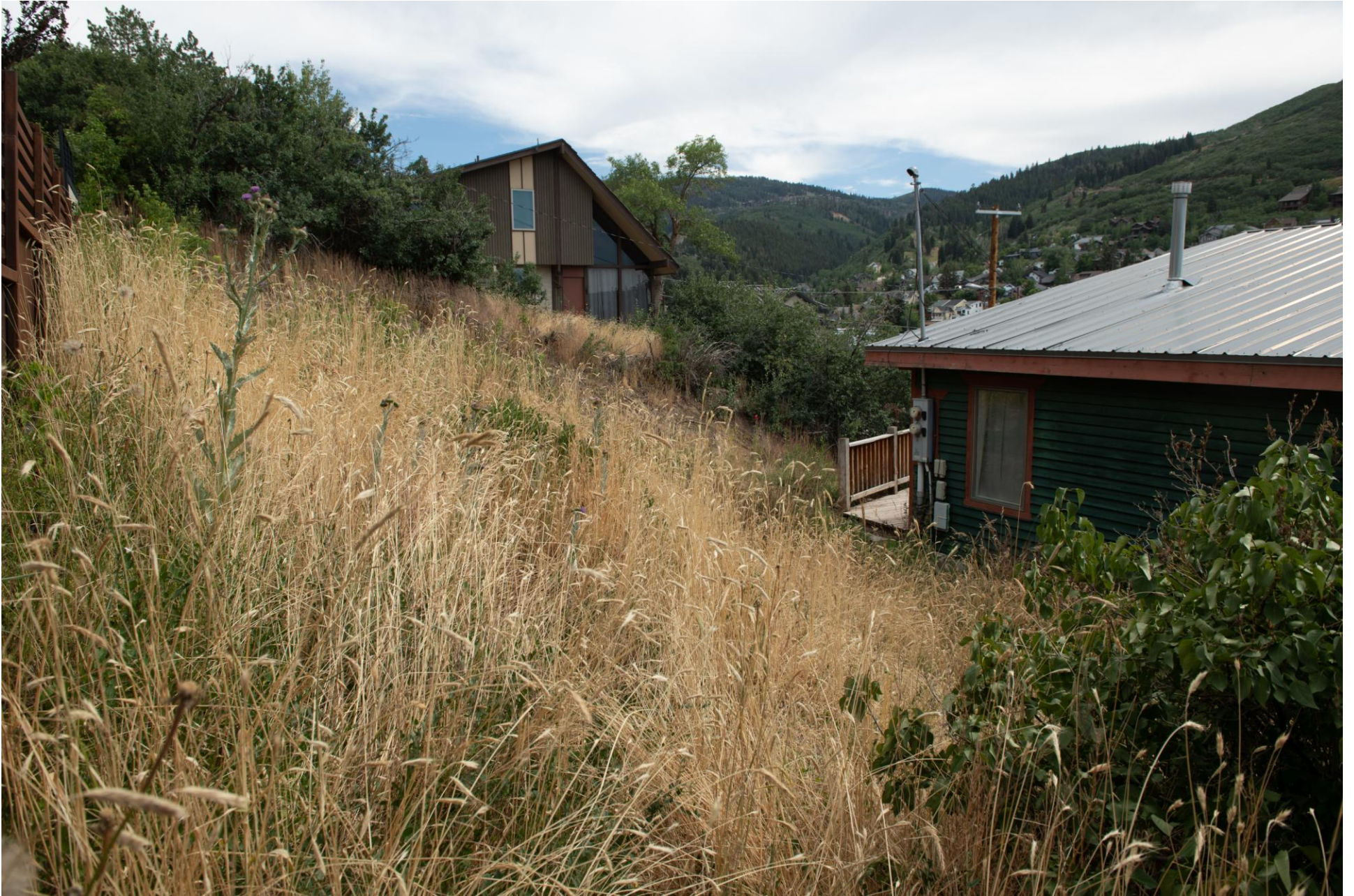
402 and 410 Ontario - rear - looking southerly
