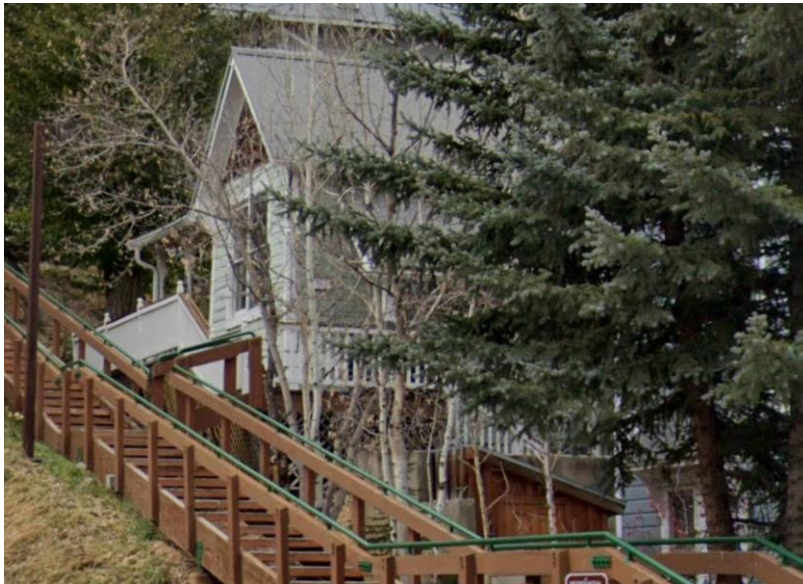
Historic Front Facing Facade along the 3 rd Street Right-of-Way viewed from Park Avenue
