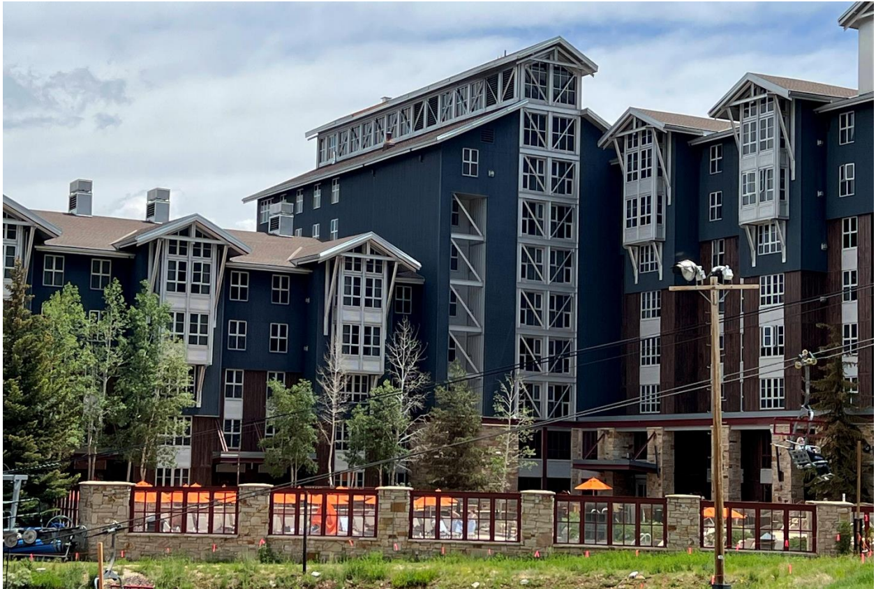
Figure 1: Marriott Mountainside Penthouse - Proposed Antenna Location
