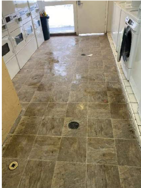
Photo 10. Holiday Village Apartments: Laundry facility.
