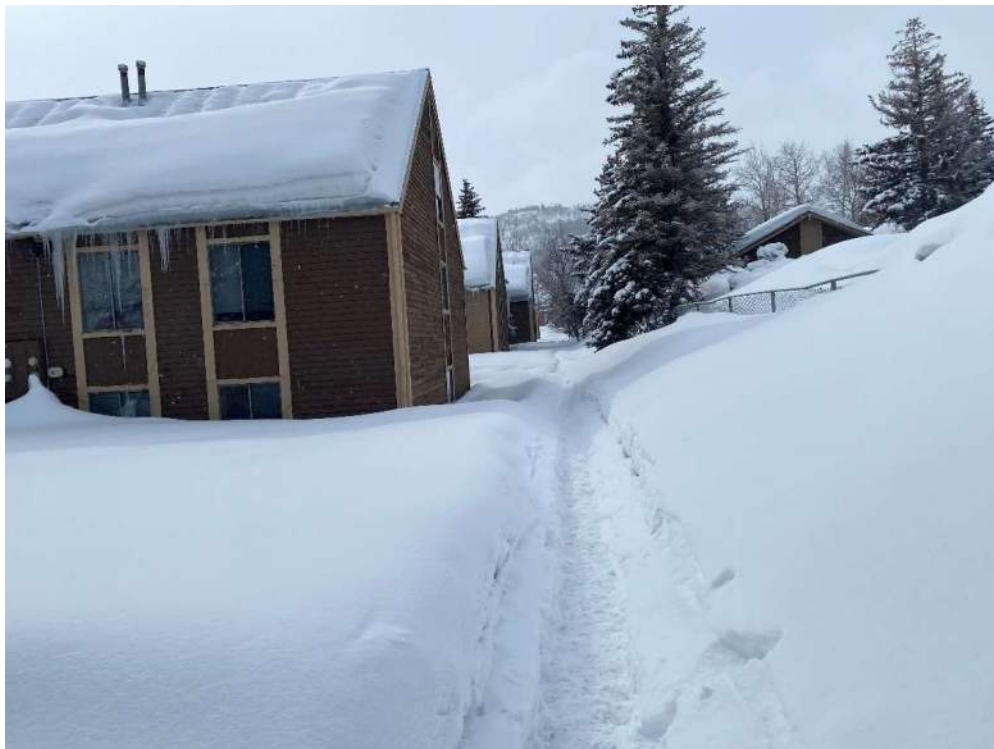
Photo 4. Parkside Apartments: Northwest corner looking south.
