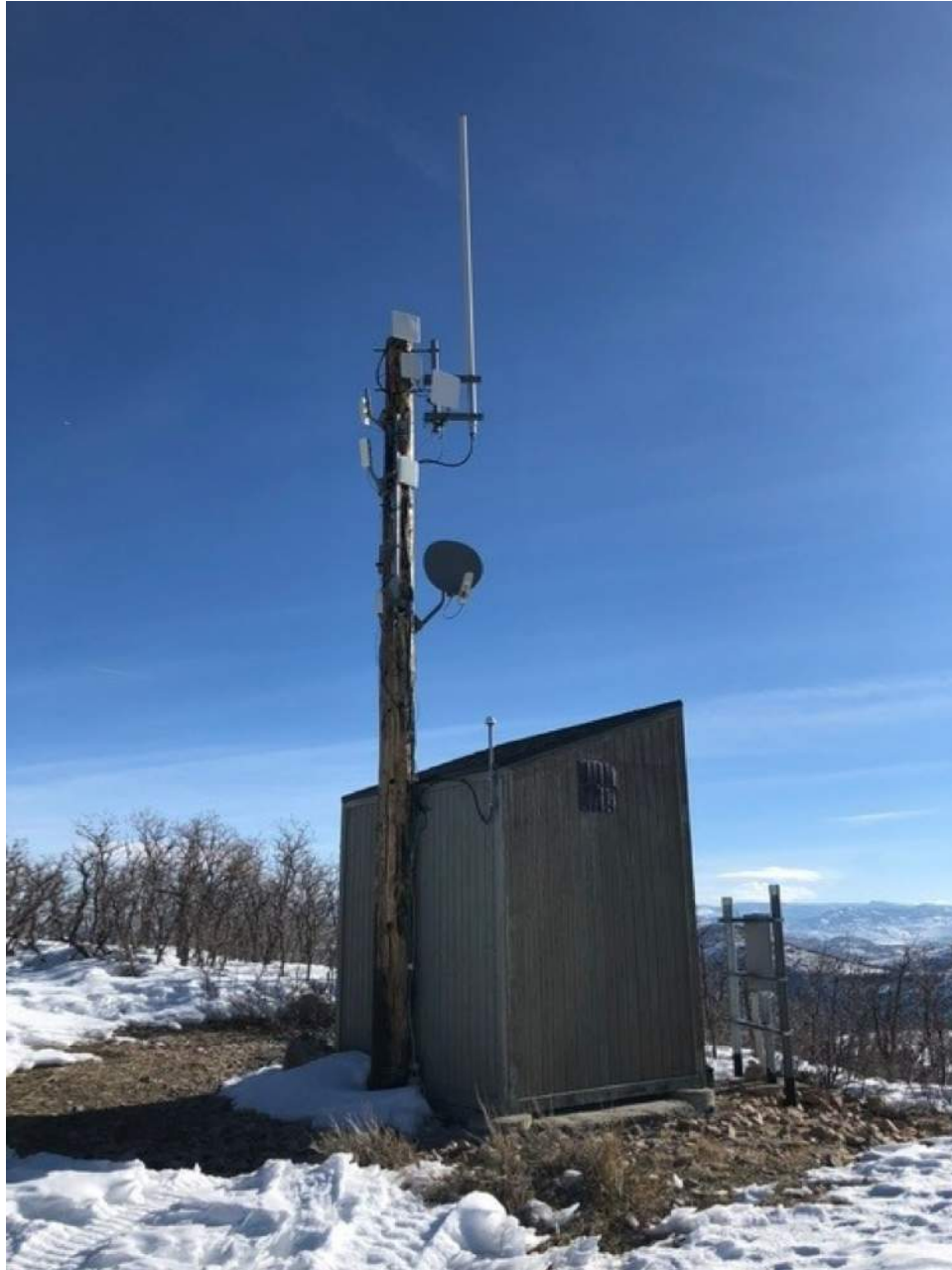
EXISTING AERIE COMMUNICATIONS TOWER & STRUCTURE TO BE REMOVED UPON COMPLETION OF NEW STRUCTURE AND INSTALLATION OF NEW RADIO EQUIPMENT
