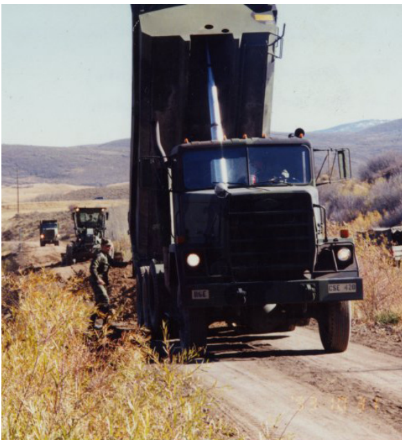
Construction of the Rail Trail
