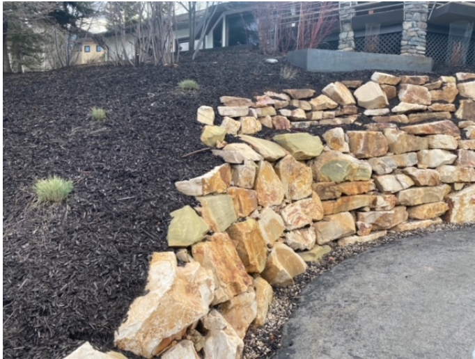
Figure 1 - Rock Wall at Entry
