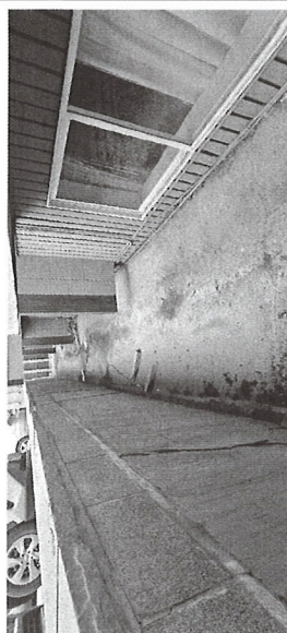
FIGURE 3: LOOKING ALONG THE WESTERN SIDE OF THE BUILDING, CONCRETE RETAINING WALL IS ON THE LEFT. CONCRETE SLAB BETWEEN THE BUILDING AND THE WALL SHOWS WITH SEEPAGE HERE
