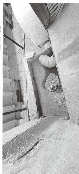
FIGURE 3: LOOKING ALONG THE WESTERN SIDE OF THE BUILDING, CONCRETE RETAINING WALL IS ON THE LEFT. CONCRETE SLAB BETWEEN THE BUILDING AND THE WALL SHOWS WITH SEEPAGE HERE
