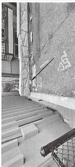
FIGURE 2: EXISTING SQUARE PORT IN THE RETAINING WALL FOR PARKING LOT DRAINAGE
