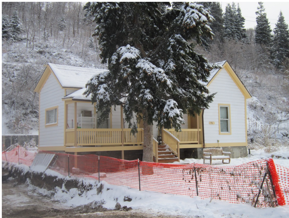
71 Daly Avenue. Northwest oblique. November 2013.
