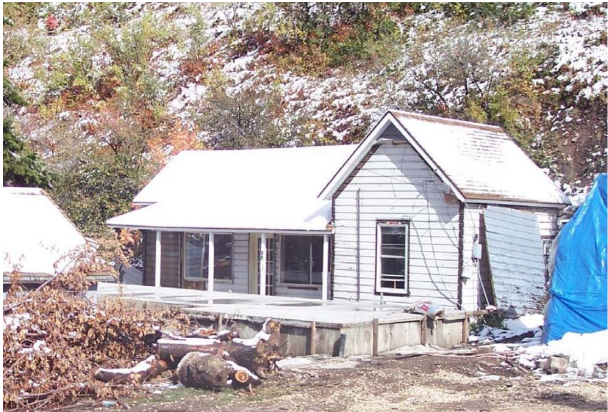
Figure 2: 71 Daly Avenue c. 2005-2006 showing new foundation prior to relocation of Structure.
