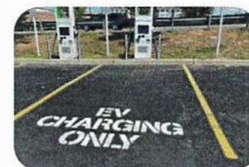
EV Charging Spaces
