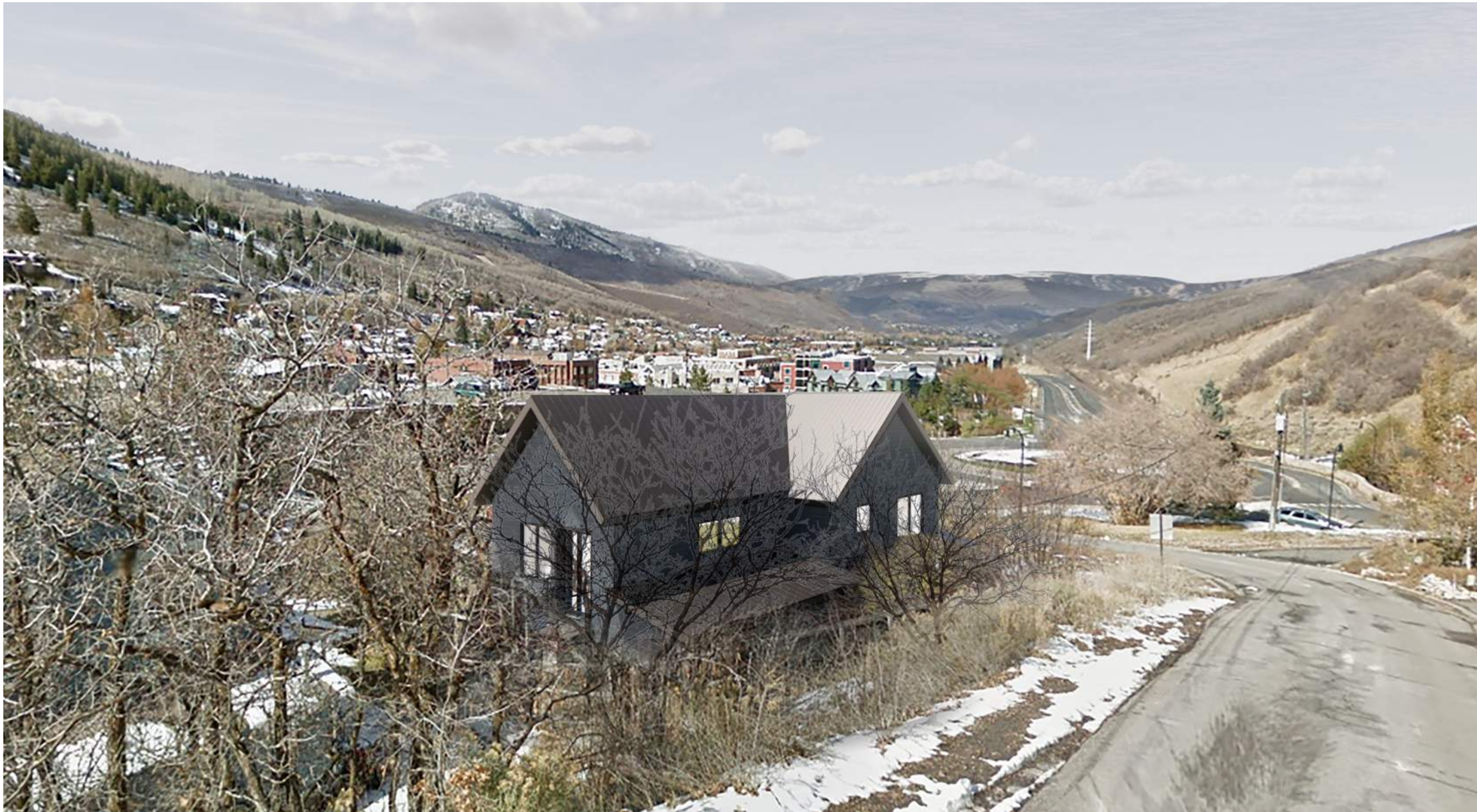
3 A005 VIEW FROM ONTARIO - SOUTH
