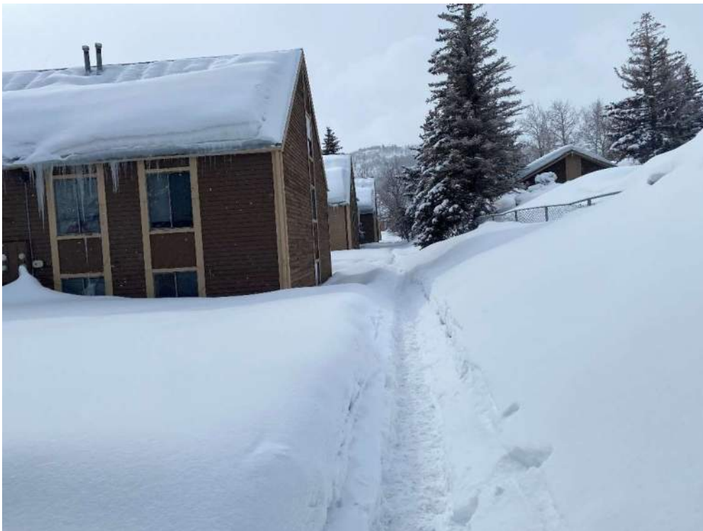
Photo 4. Parkside Apartments: Northwest corner looking south.
