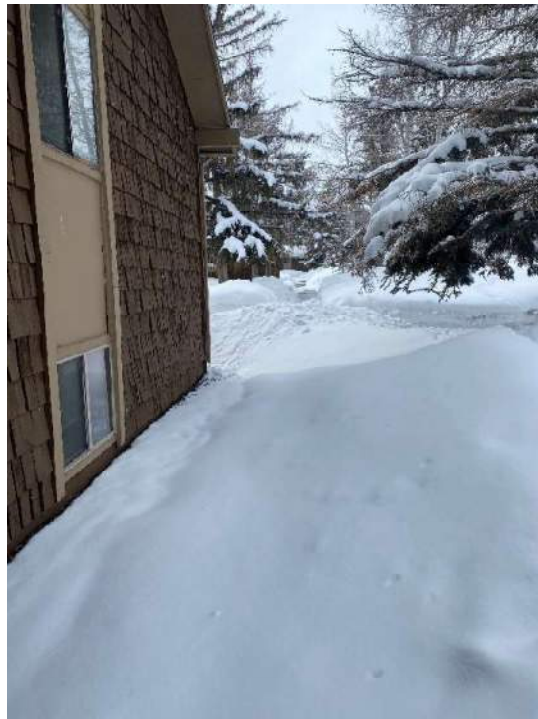
Photo 7. Holiday Village Apartments: Northwest corner looking south.
