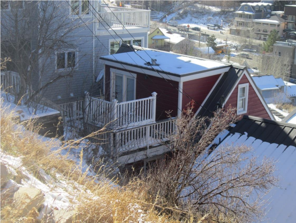
317 Ontario Avenue. Northeast oblique. November 2013.
