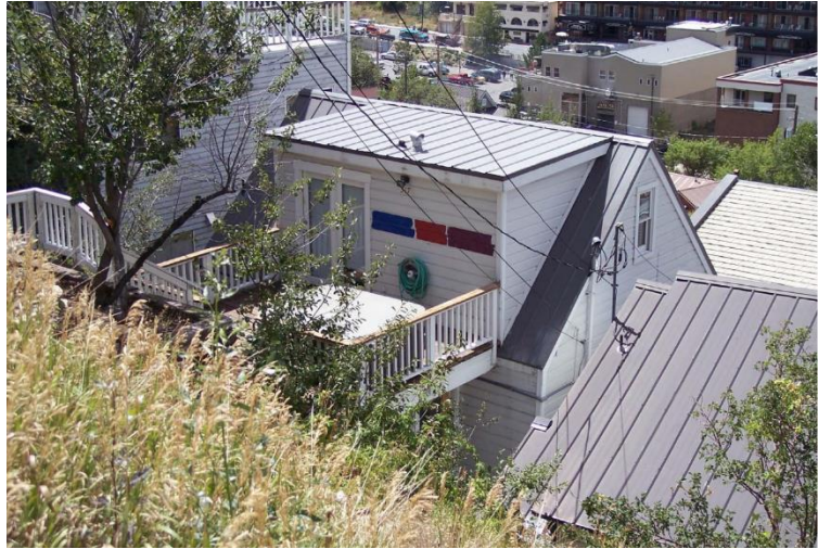
Figure 2: View of rear showing modified roof form and balcony
