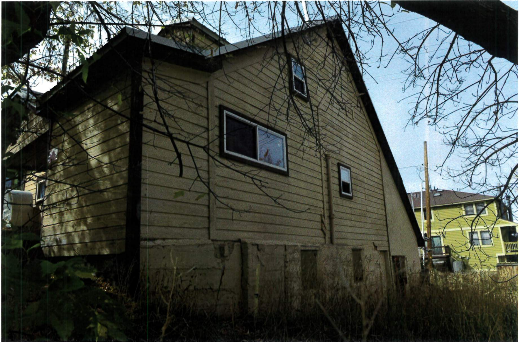
844 Empire Avenue looking northwesterly
