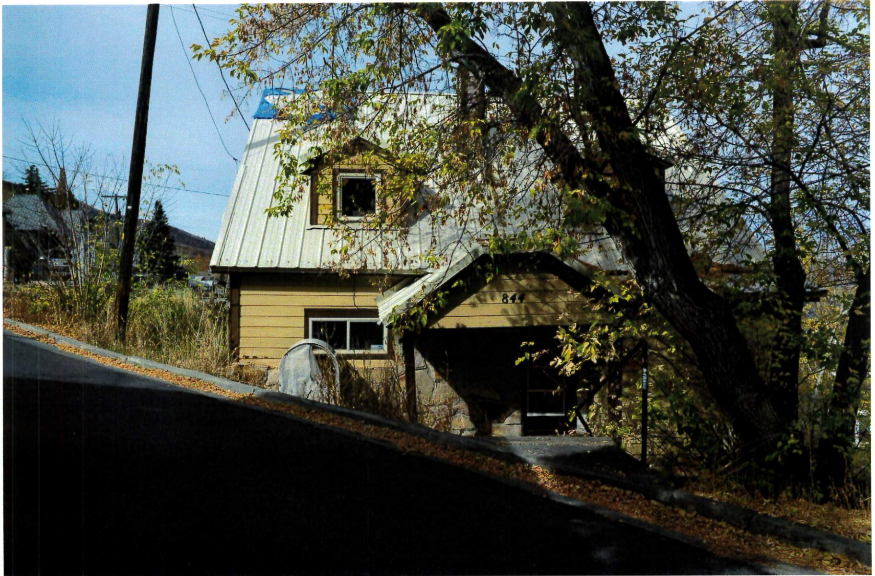
844 Empire Avenue looking northerly
