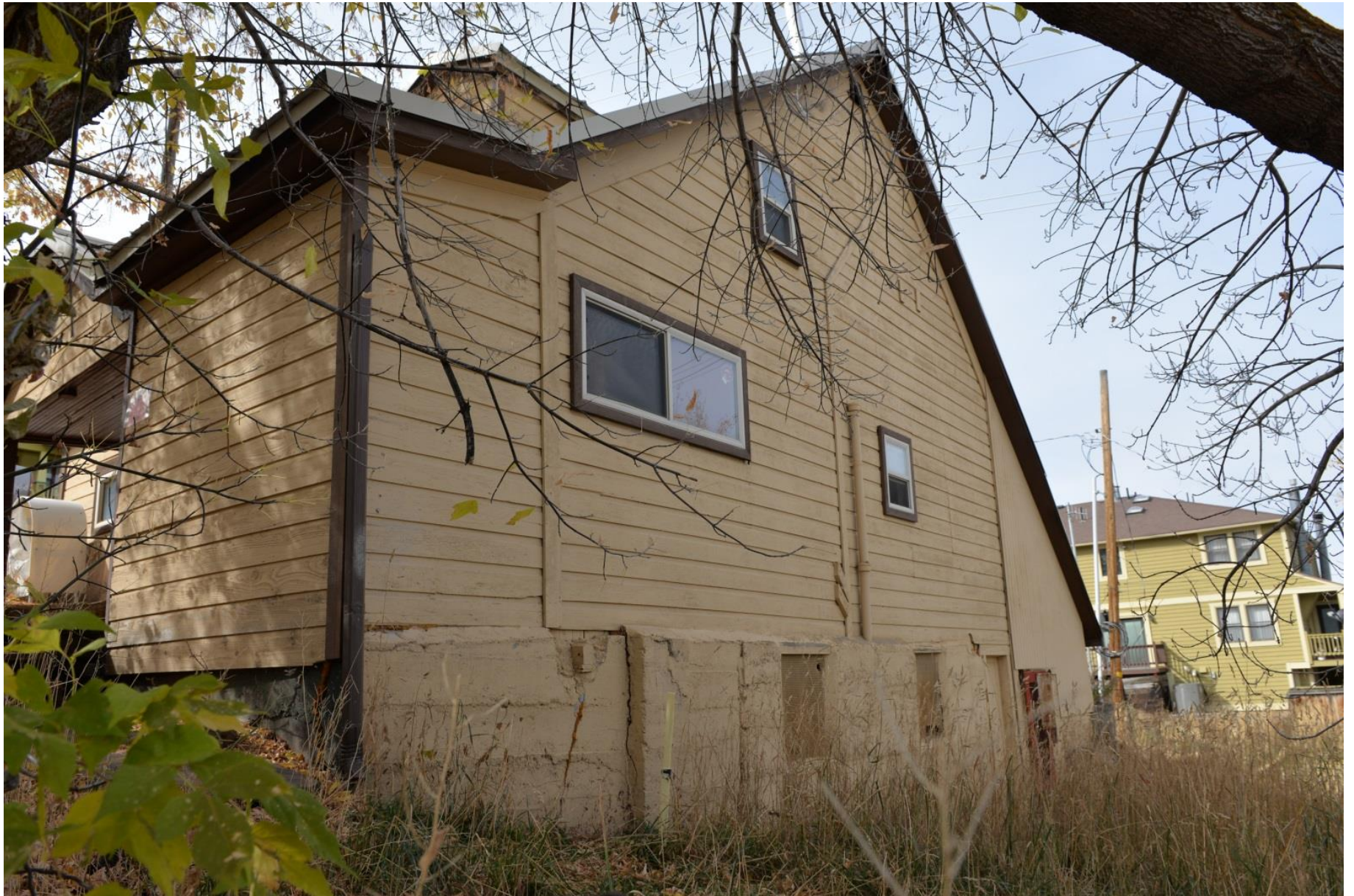
844 Empire Avenue looking northwesterly
