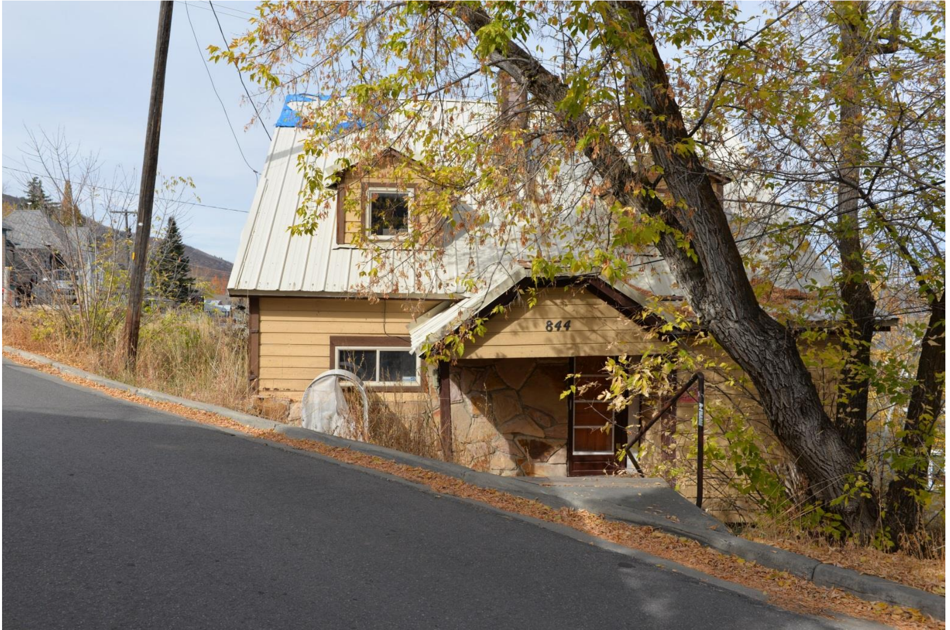
844 Empire Avenue looking northerly
