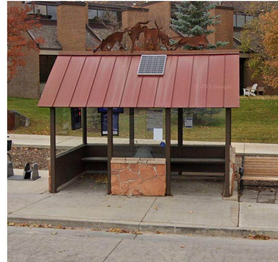
Existing Bus Stop
