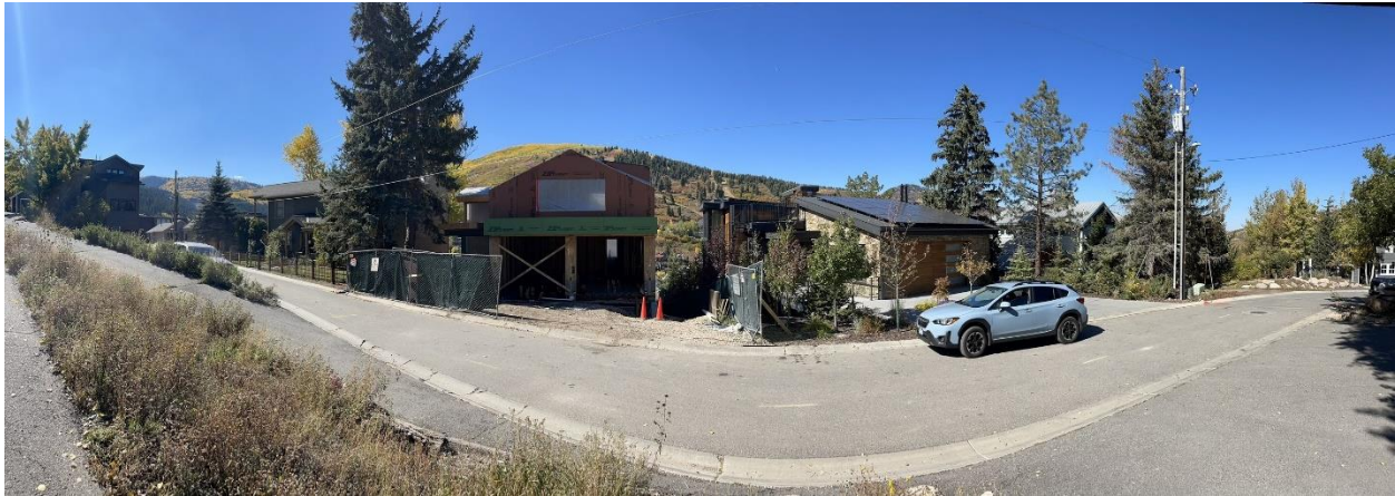
Figure 2: Street View of Front Yard from McHenry Avenue
