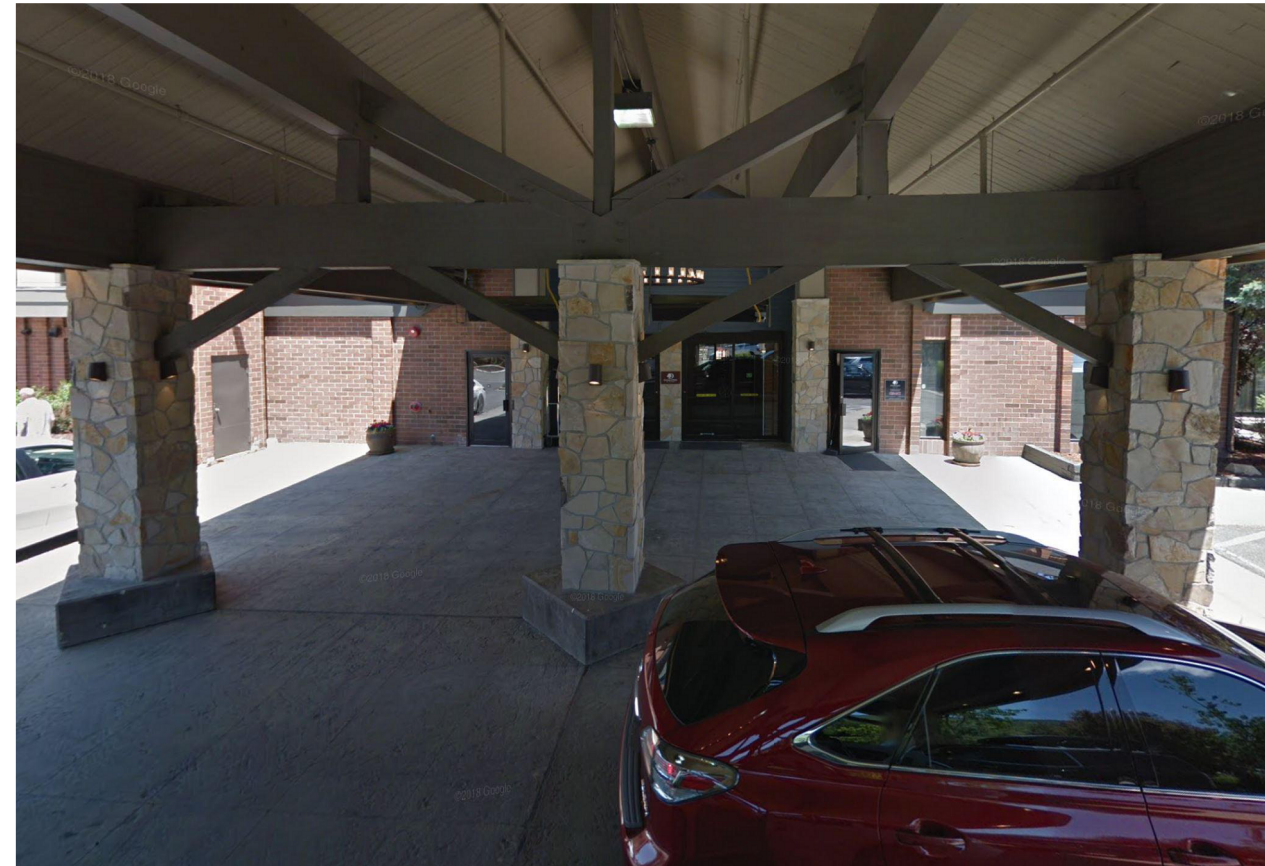
Existing Bus Stop
