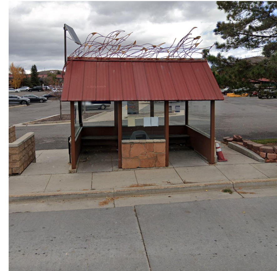
Existing Bus Stop, under Construction
