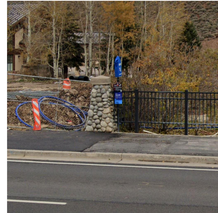
Existing Bus Stop
