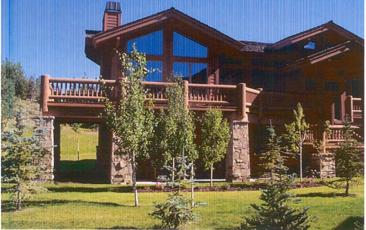
Looking north from rear of Unit 1
