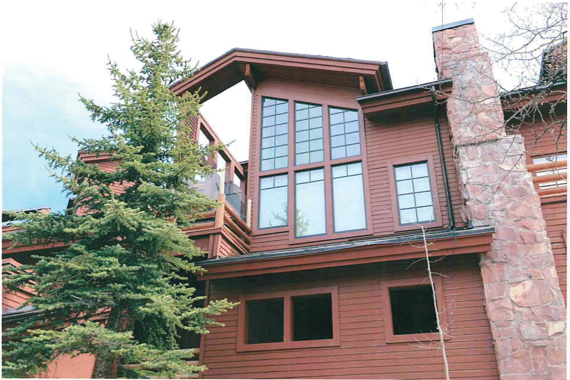
Stag Lodge, Phase 1, Unit 10
