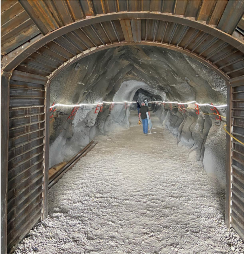
Figure 2. Inside the Spiro Tunnel, October 2021
