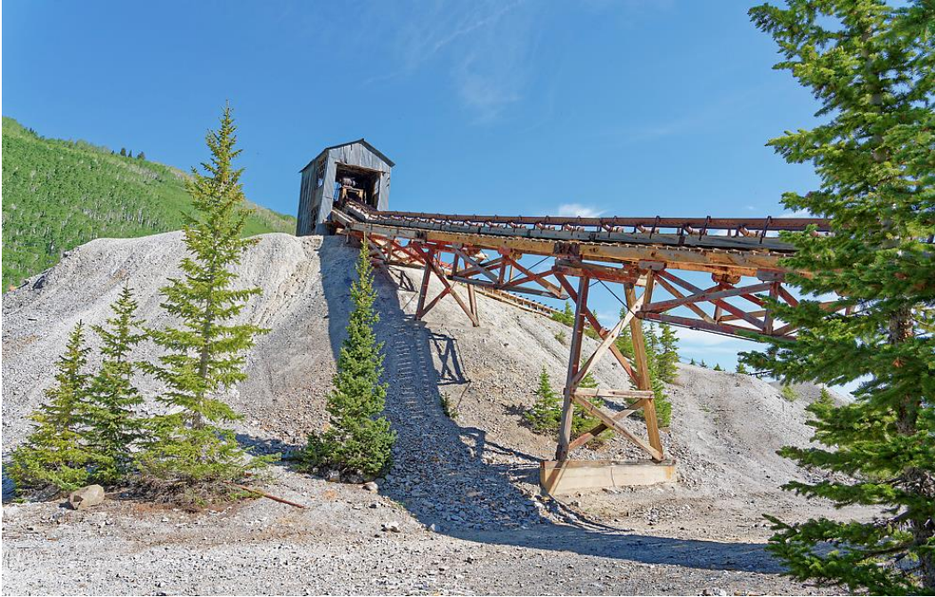
Figure 4. Thaynes Conveyer Gallery, 2021
